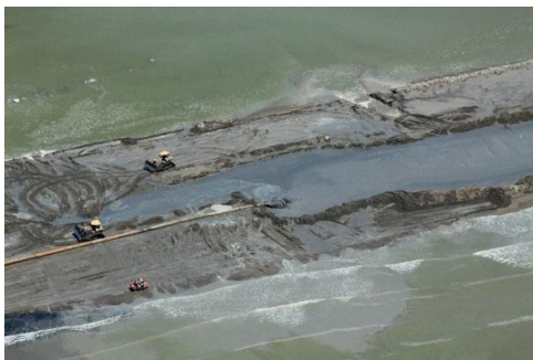
W9 Berm Operations – September 9, 2010
