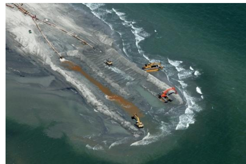
E4 North Berm – September 9, 2010
