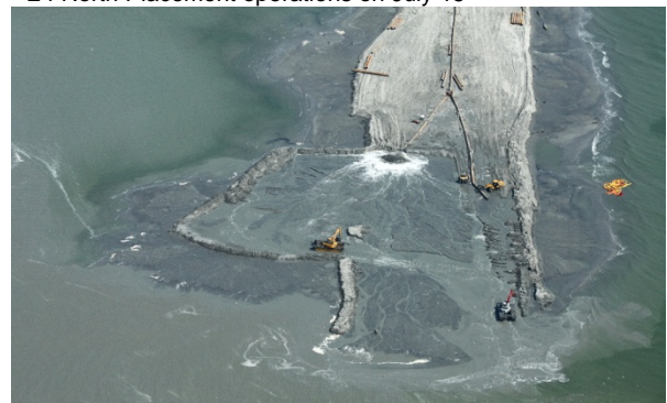
*Continued E4 Berm Placement
