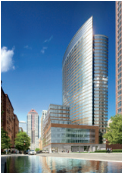
The Visionaire, shown here in an artist's rendering, is a luxury green condominium tower in New York City.
