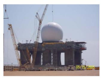
PHOTO CAPTION: The SBX radome provides the characteristic "radar" silhouette after being installed over the weekend.
