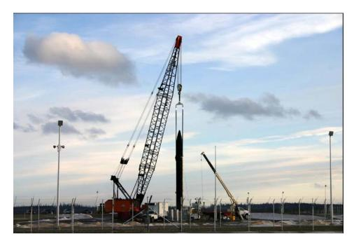
PHOTO CAPTION: The sixth Ground-based Interceptor missile is lowered into its underground silo at Ft. Greely, Alaska on November 11, 2004. The interceptor is part of a missile defense system designed to intercept and destroy a long-range ballistic missiles. Although the system will have a limited initial capability, it will be the first time the United States will have a missile defense system to protect all 50 states.
