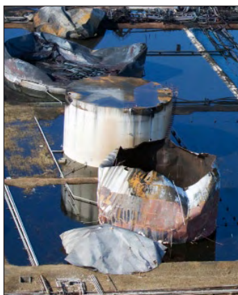
Wreckage of fuel tanks near Fort Buchanan.
