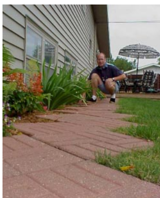
Terry Styf installed pavers with a slight angle to drain water away from his house.
