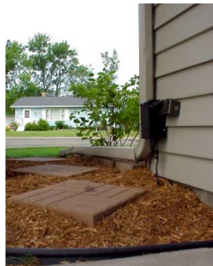
More pavers outside Styf's garage also help direct water away from the structure and foundation.
