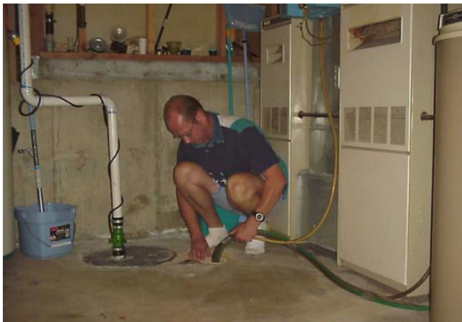
Styf secures hoses into a basement drain.
