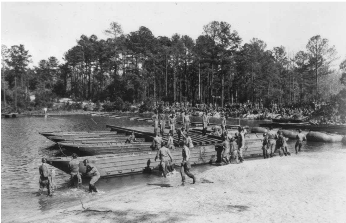
Figure 66. Aluminum balk pontoon bridge construction on Smith Lake at Fort Bragg, NC, 1951 (NARA College Park, RG 111-SC WWII, Box 207, Photo SC370521).
