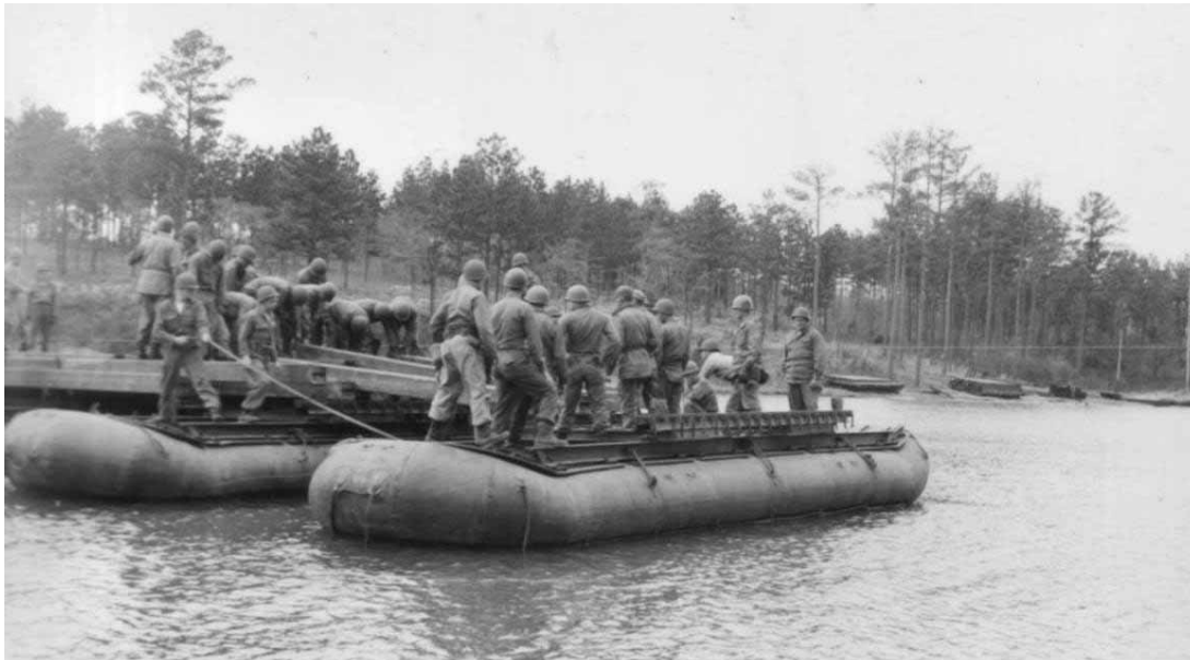
Figure 67. Engineers building a heavy equipment bridge across Smith Lake at Fort Bragg, NC, 1 April 1951 (NARA College Park, RG 111-SC WWII, Box 212, Photo SC376463).
