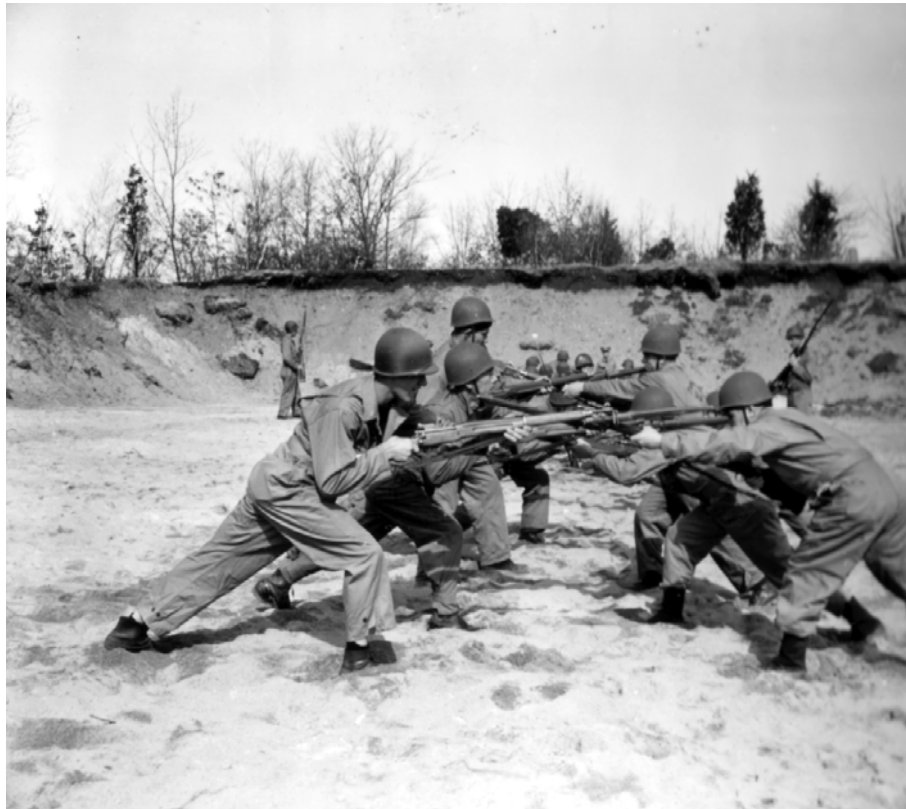
Figure 1. Seabees during bayonet training at Camp Endicott, Davisville, RI, May 1943 (NARA College Park, RG 80-G, Box 172, Photo 38061).
