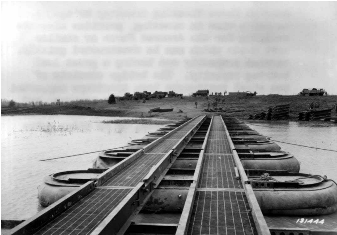
Figure 65. A floating treadway bridge at Fort Knox, KY, April 1942 (NARA College Park, RG 111-SC WWII, Box 42, Photo SC131444).
