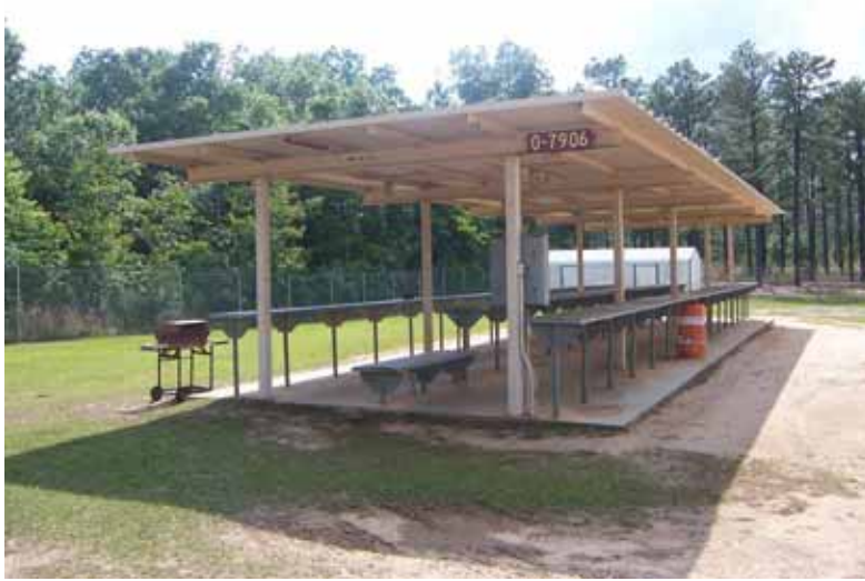
Figure 351. Range mess facilities O-7906, Fort Bragg, 17 May 2006.
