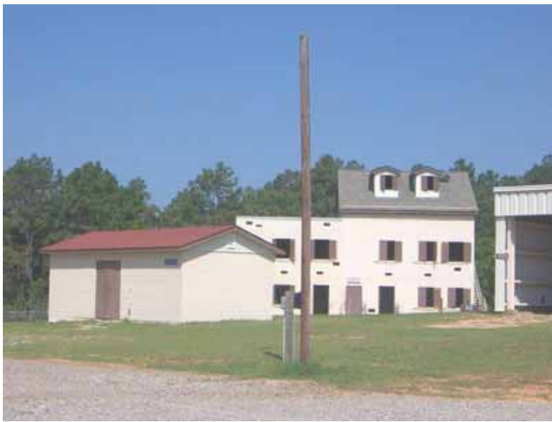
Figure 333. Range storage building, Fort Bragg, 17 May 2006.
