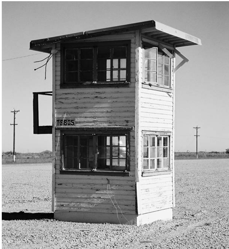
WWII Observation tower Bldg 9805, Fort Bliss, TX, November 2005.
