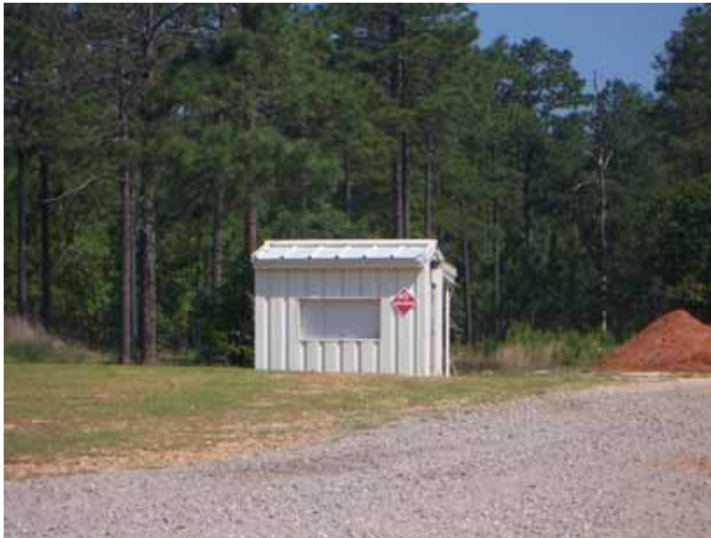
Figure 334. Range storage building, Fort Bragg, 17 May 2006.
