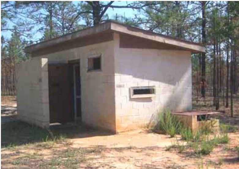
Figure 343. Range latrine, Fort Bragg, 17 May 2006.
