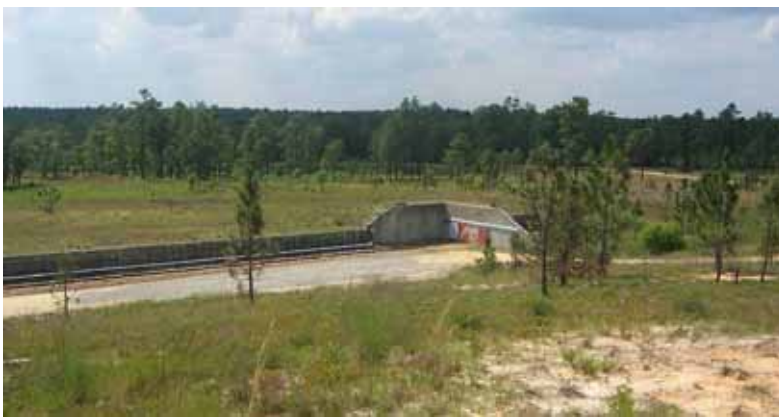
Figure 302. Target storage and repair building at the end of the target track protected by an embankment, Fort Bragg, 17 May 2006.
