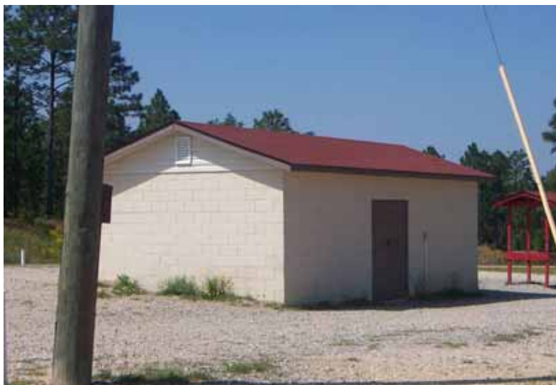
Figure 331. Range storage building, Fort Bragg, 17 May 2006.
