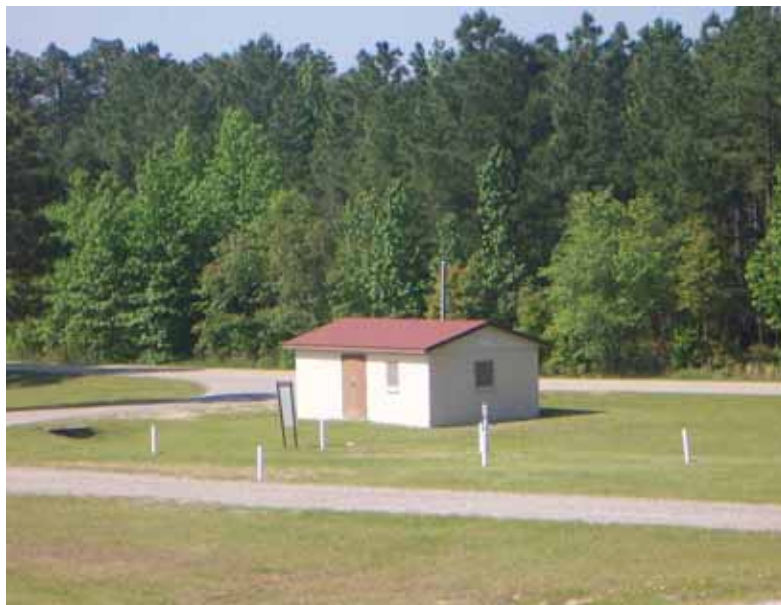
Figure 330. Range storage building, Fort Bragg, 17 May 2006.
