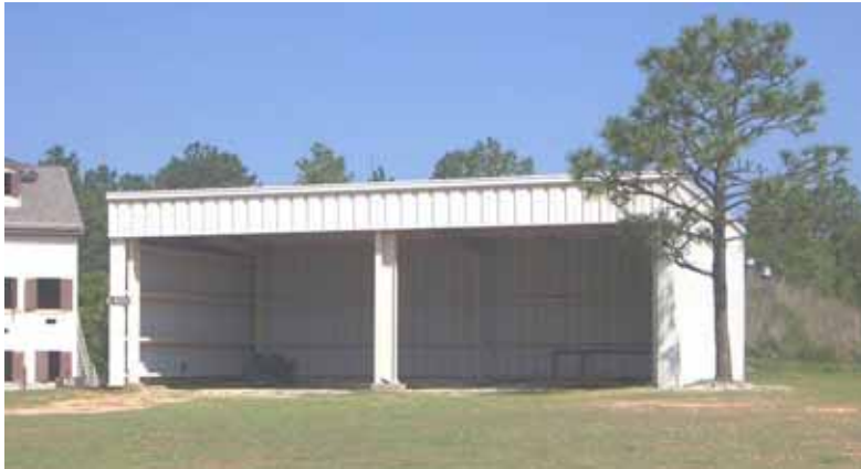
Figure 332. Range storage building, Fort Bragg, 17 May 2006.
