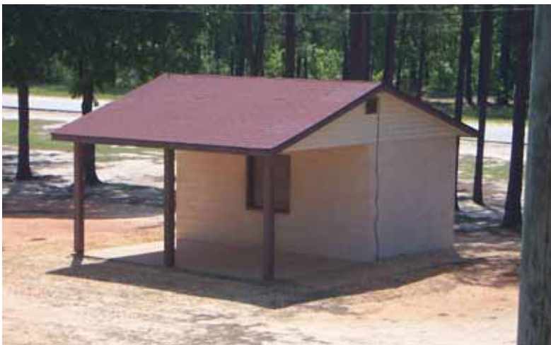
Figure 337. Range ammunition storage building, Fort Bragg, 17 May 2006.
