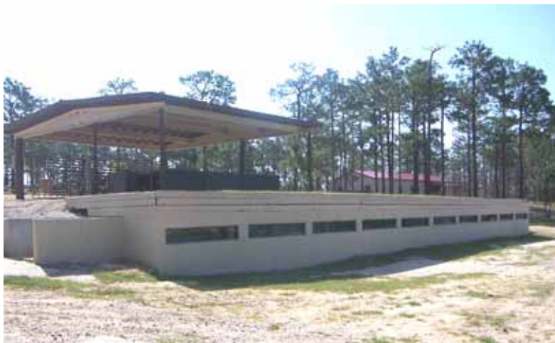
Figure 348. Range bleachers, Fort Bragg, 17 May 2006.
