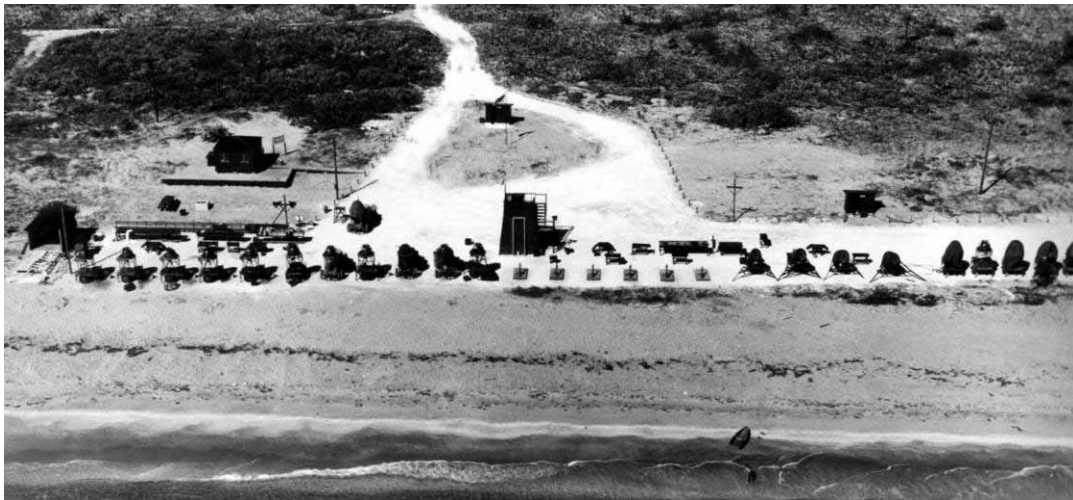
Figure 108. Beach firing range at NAS Fort Lauderdale, FL, 28 February 1944 (NARA College Park, RG 80-G, box 1513, photo 388275).
