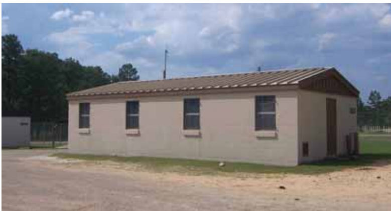
Figure 328. Range storage building, Fort Bragg, 17 May 2006.
