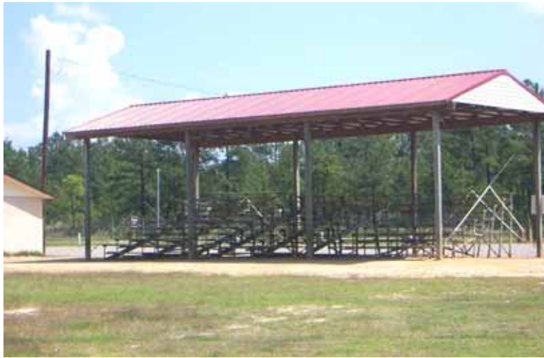
Figure 346. Range bleachers, Fort Bragg, 17 May 2006.
