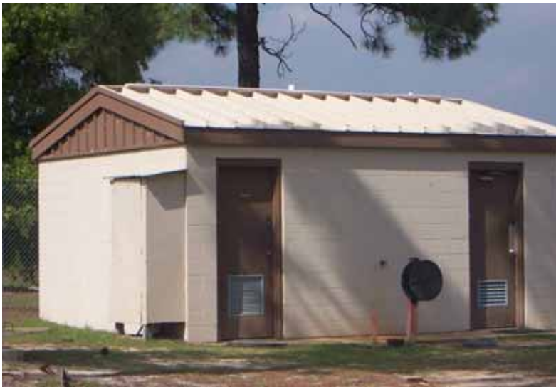
Figure 344. Range latrine, Fort Bragg, 17 May 2006.
