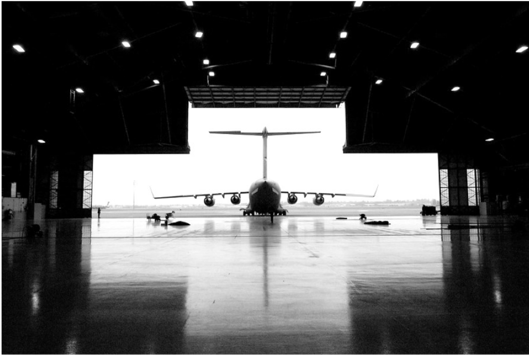
FIGURE 5-10. HANGAR WITH CANOPY DOOR TAIL CUT AT WRIGHT PATTERSON AFB
