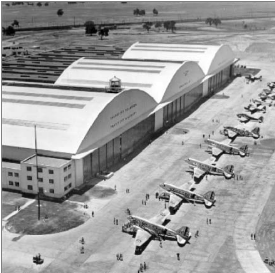
FIGURE 4-16. THREE-ARCH HANGAR, MCCLELLAN FIELD, CALIFORNIA, LATE 1930S
