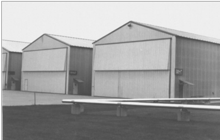
FIGURE 5-9. CANOPY HANGAR DOORS AT DES MOINES ANG BASE
