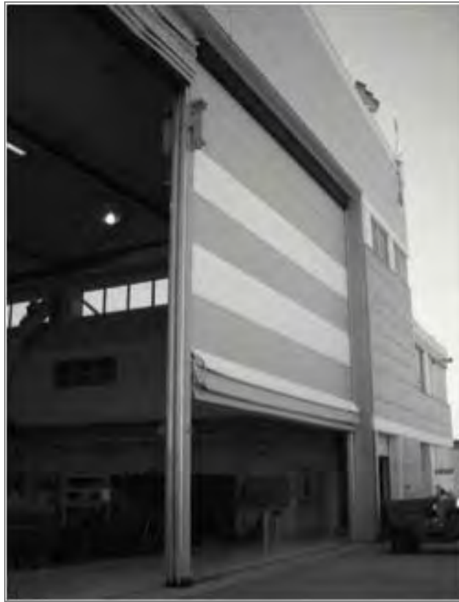
FIGURE 5-8. DETAIL OF CANOPY HANGAR DOOR AT OHIO ANG BASE IN TOLEDO, OHIO
