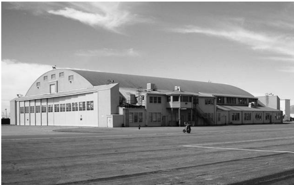
FIGURE 5-7. MULTILEAVED DOORS ON HANGAR AT BIGGS ARMY AIRFIELD, EL PASO, TEXAS
