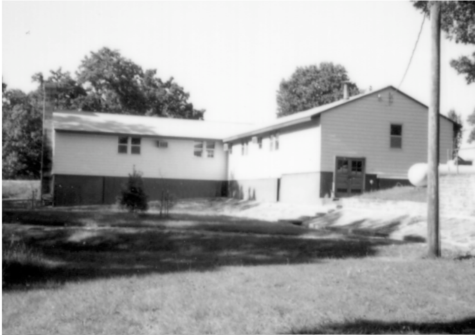
Figure 4.8 Building 2101 From Ravine (SCIAA).
