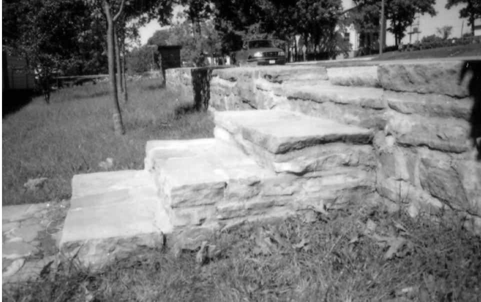
Figure A-3 POW Stonework Steps, Building 2101 (SCIAA).
