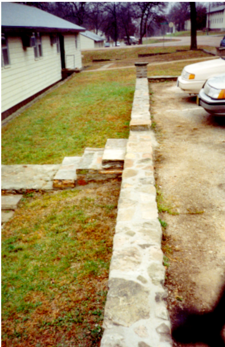
Figure A-2 Restored Wall In Front of Building 2101 (Courtesy USACERL).
