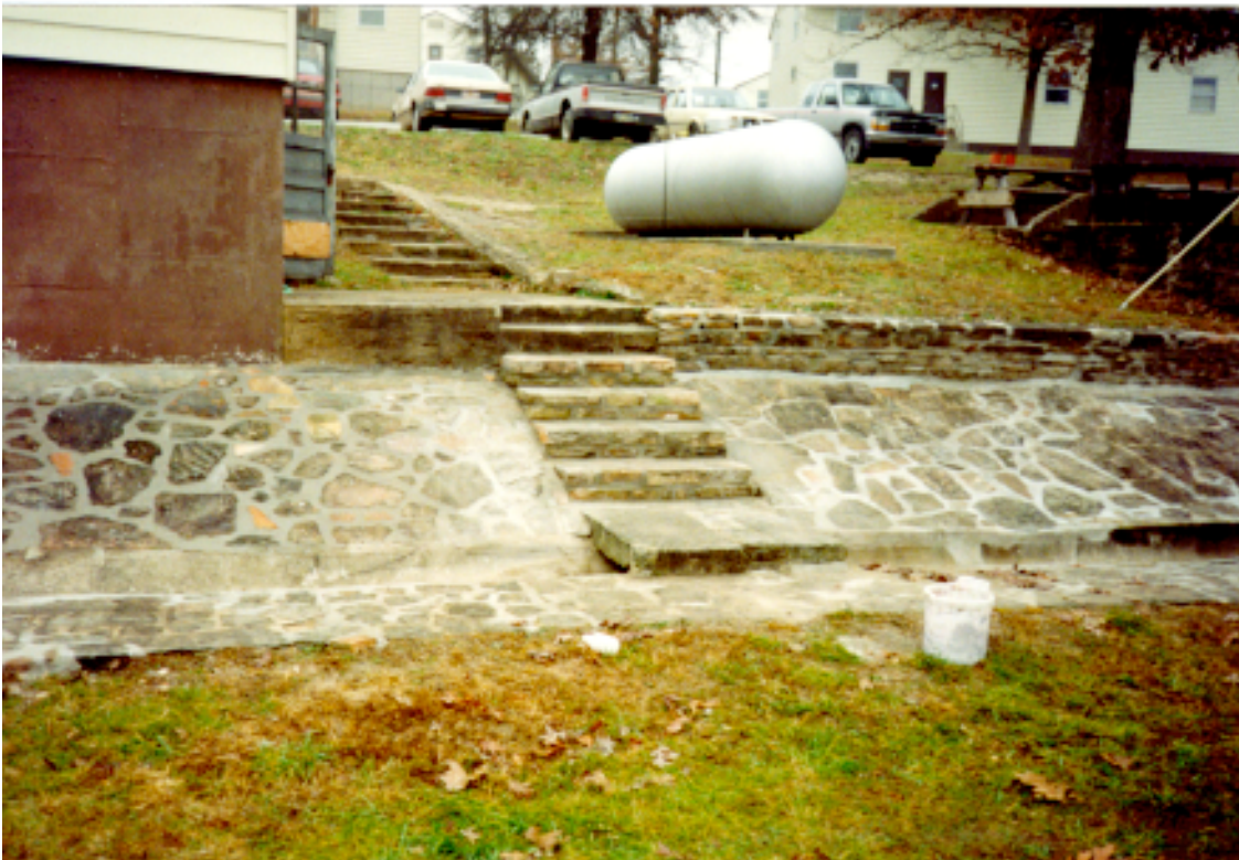
Figure A-1 Stone Steps, Retaining Walls After Restoration, Building 2101 (courtesy USACERL).
