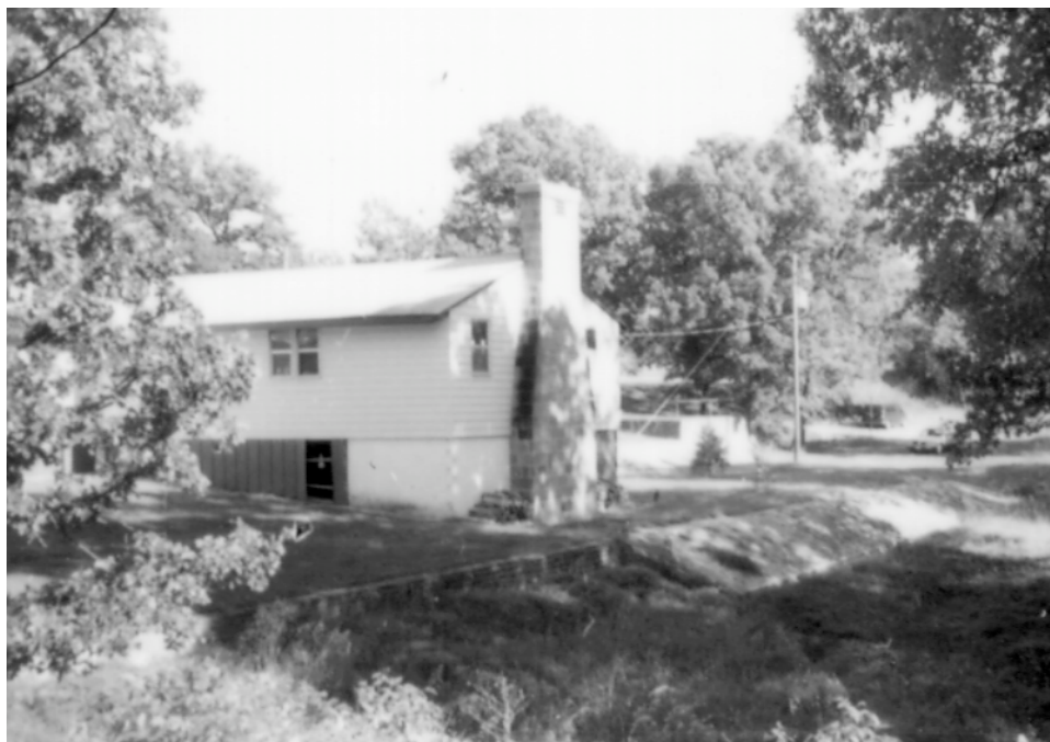
Figure 4.9 Building 2101, Rear From Street (SCIAA).
