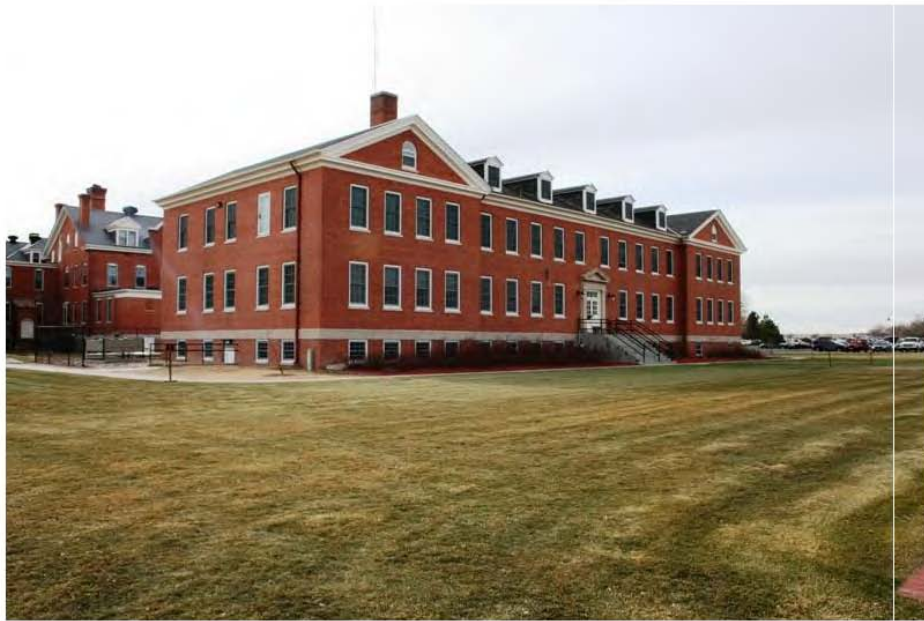
Medical Detachment Barracks, Building 152, view to southwest
