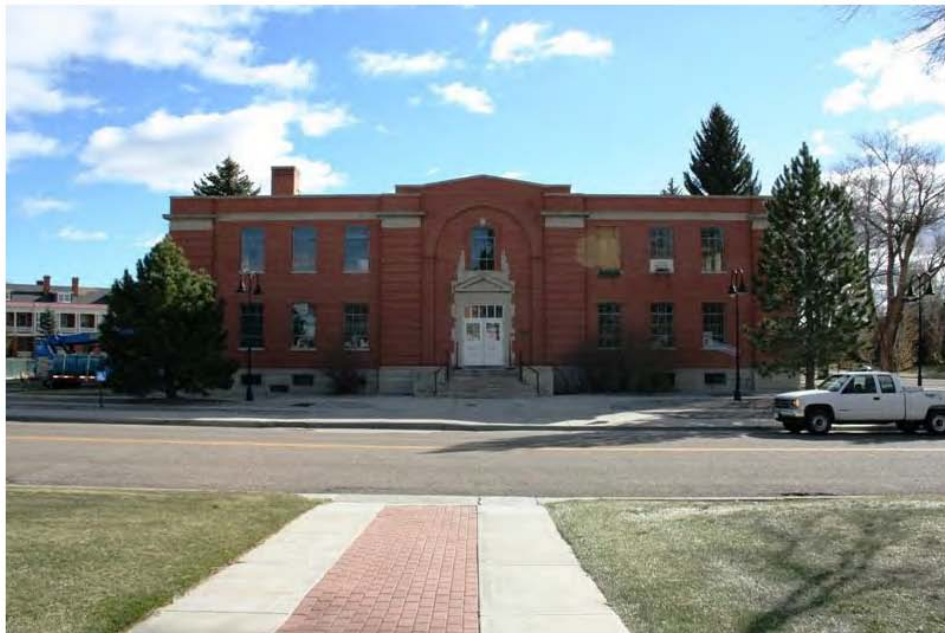
Base Gym, Building 151, view to east
