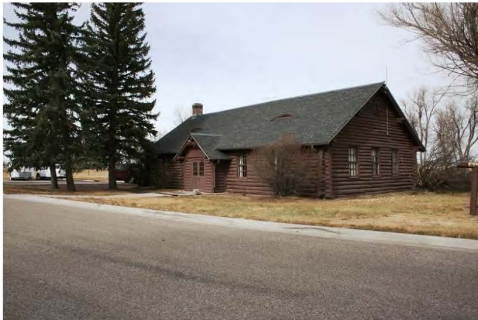
Boy Scout Lodge, Building 153, view to northwest
