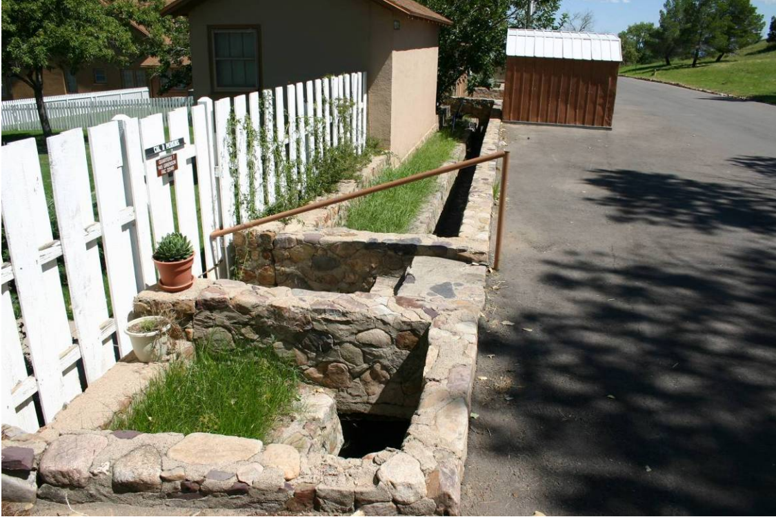
Figure 4-10. Ditches along Grierson Street
