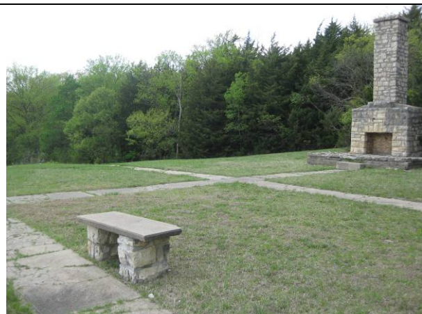
Figure 4-13: Foundation with sidewalks, bench and rebuilt fireplace/chimney.
