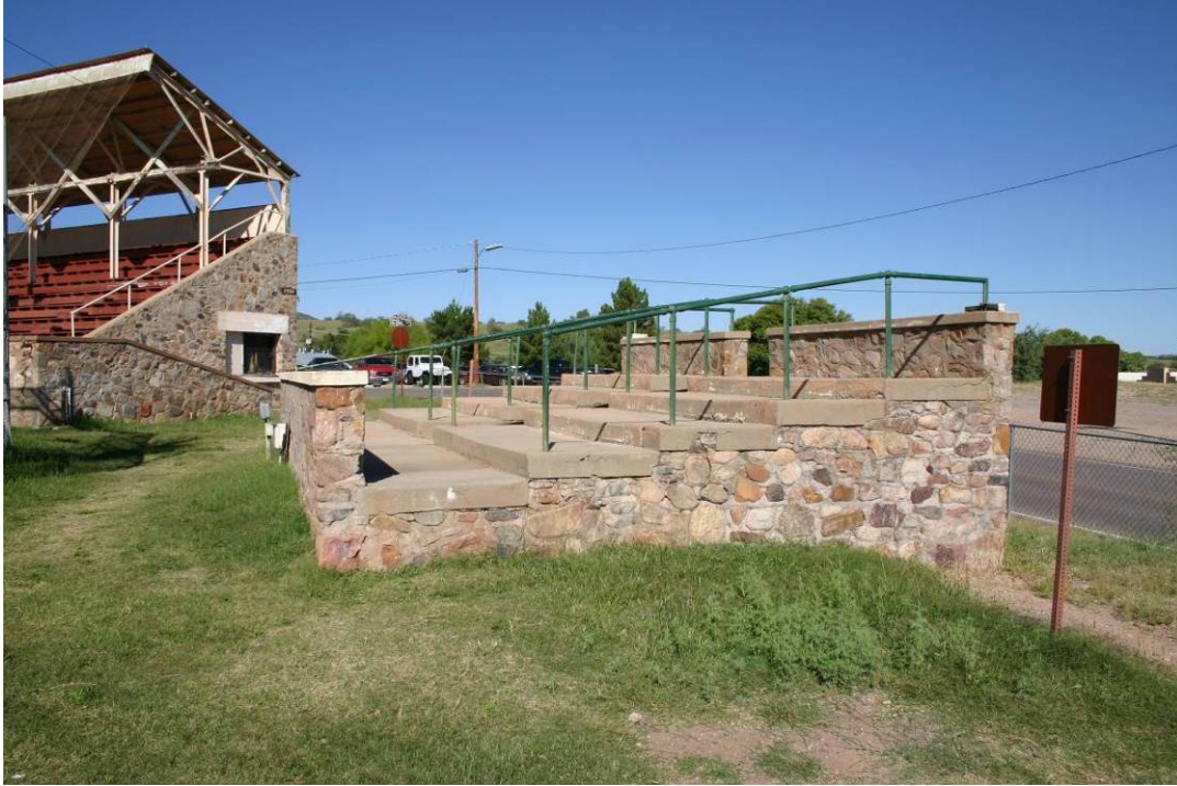
Figure 4-5. Officers' Grandstand (31123), Brock Field
