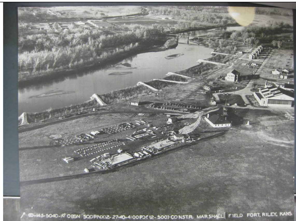
Figure 4-3: Photo of Marshall Field cantonment area showing WPA rock dikes along Kansas River, December 1940. Levee now rests along inland base of buried rock dikes. Photo courtesy of the Fort Riley Museum Archives.
