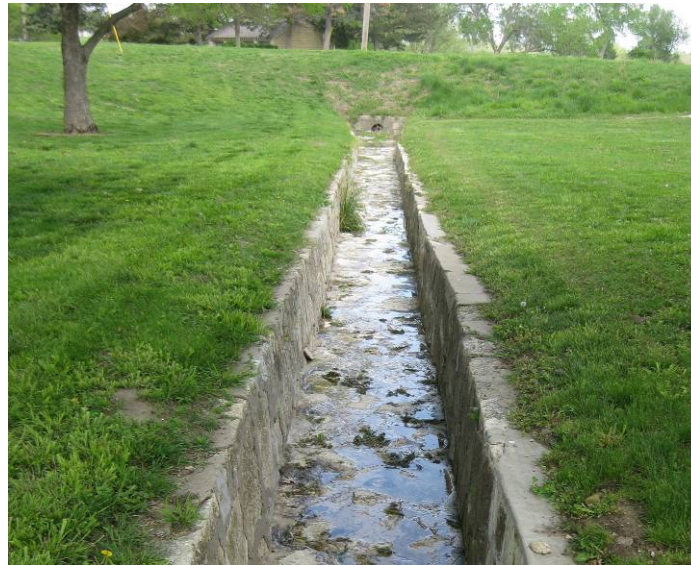
Figure 4-7: Stem of ditch which terminates in the drain under Godfrey Avenue.
