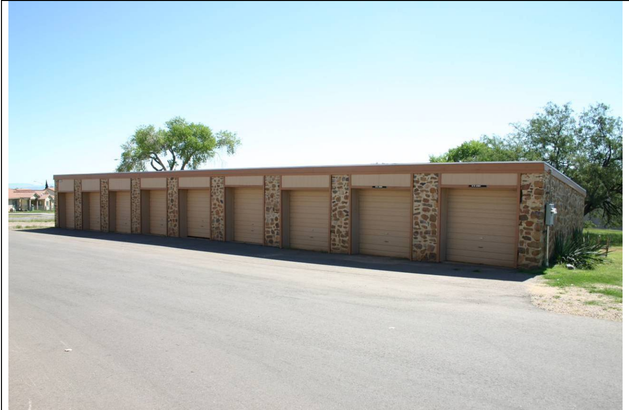
Figure 4-11. Nine bay garage (42021) behind Allen House.
