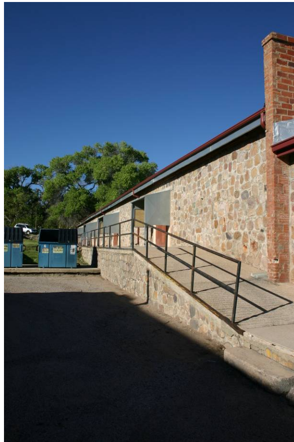
Figure 4-16. Utilities Warehouse before and after WPA renovations.
