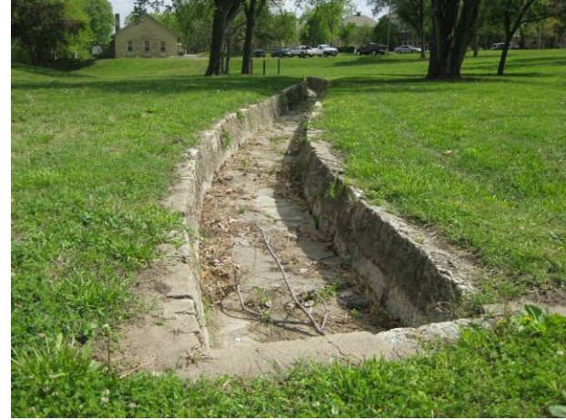
Figure 4-6: North arm of ditch. Building 430 at upper left.
