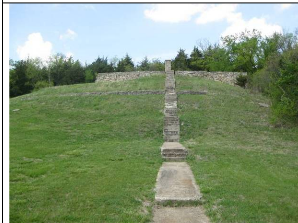
Figure 4-12: Concrete stairs to foundation. Upper terrace is visible just below foundation wall.
