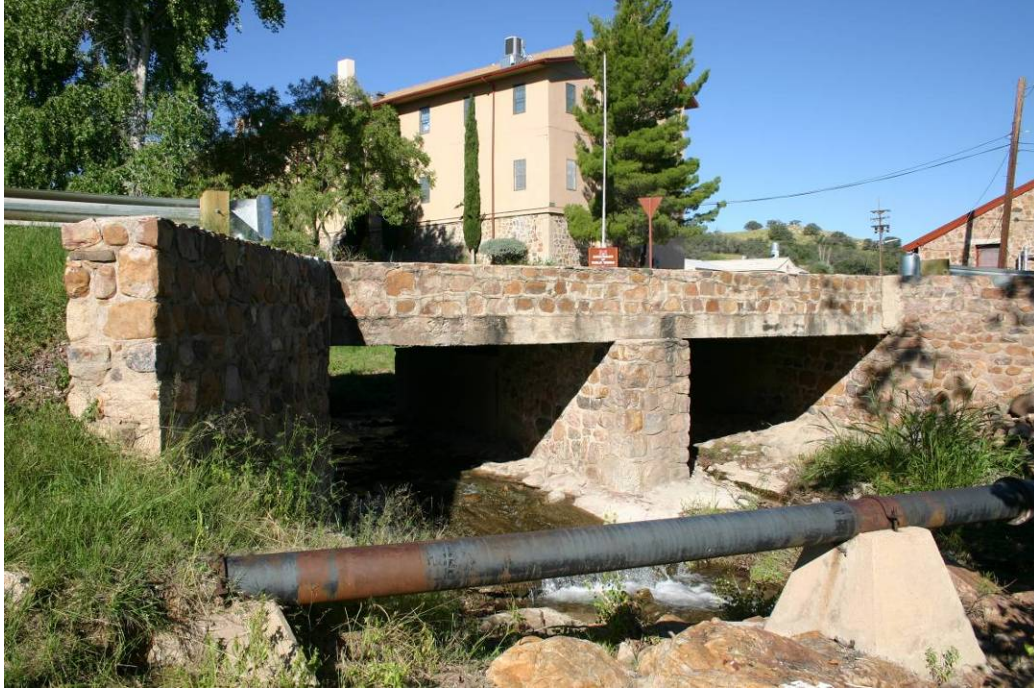
Figure 4-7. Bridge over Huachuca Creek.
