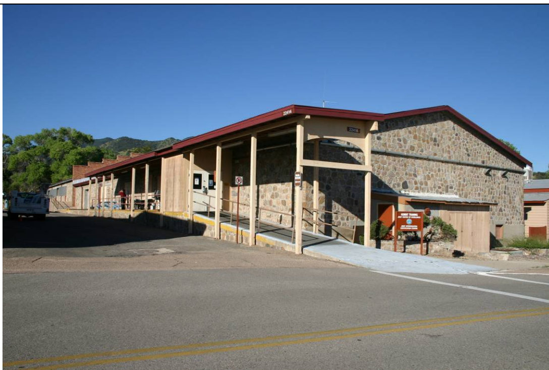
Figure 4-15. Former Utilities Warehouse (22414)
