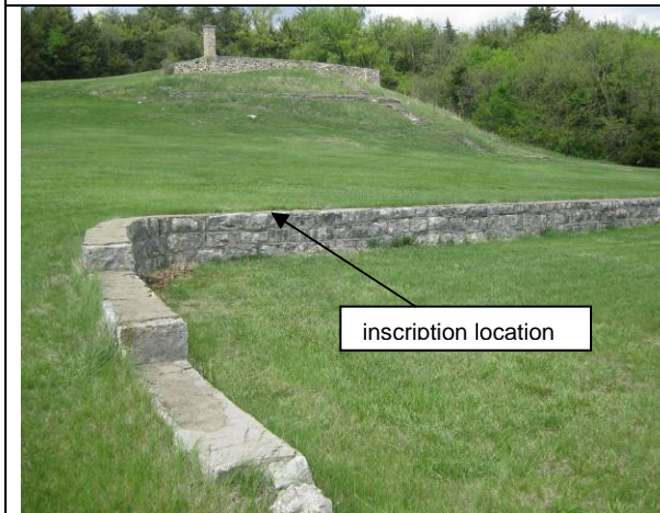
Figure 4-10: Lower terrace in foreground, upper terrace and foundation wall in background.
