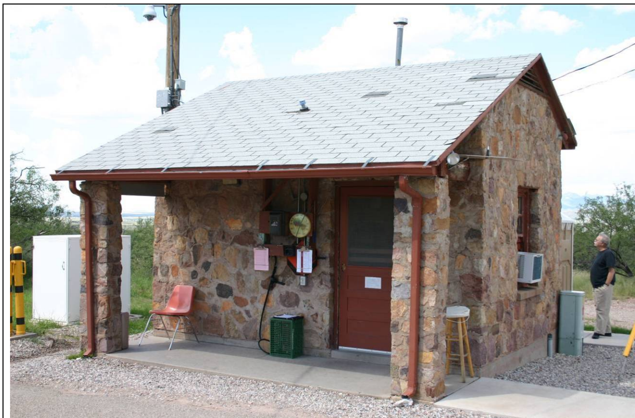
Figure 4-13. West (Canelo) Gate Guardhouse (11510)
