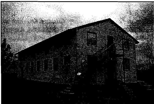
Figure 15. Building 2531 serves as a curation facility on Fort Polk.
