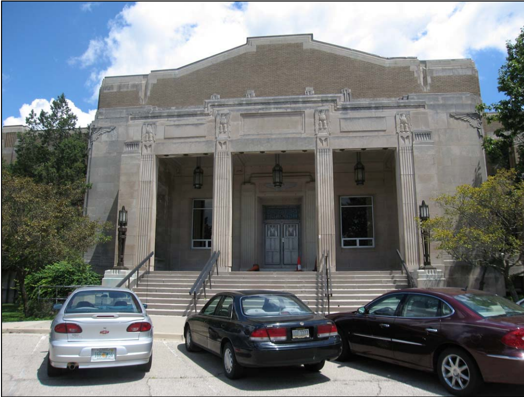
Figure 8. Building 20012 (built 1934–1935), Wright-Patterson Area B, designed by Albert and Freeman Pretzinger, view of main entrance
