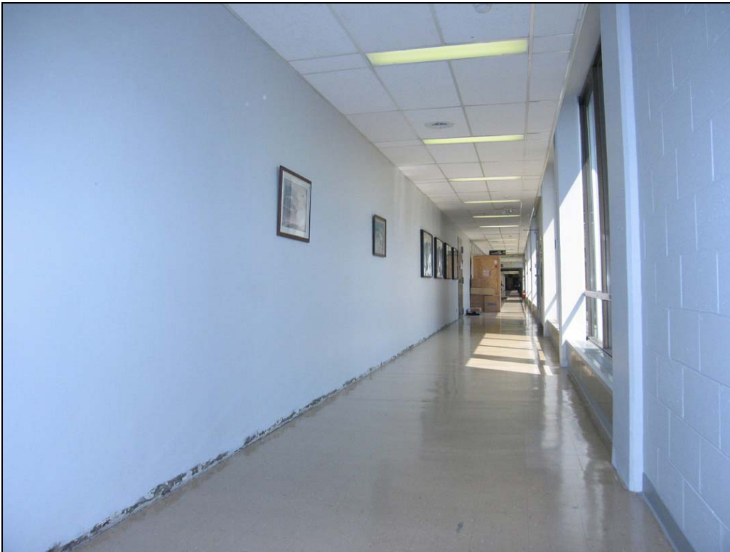
Figure 52. Building 20620, second-floor corridor
