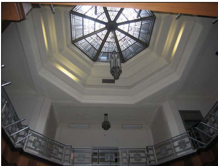
Figure 10. Building 20012, detail of interior skylight
