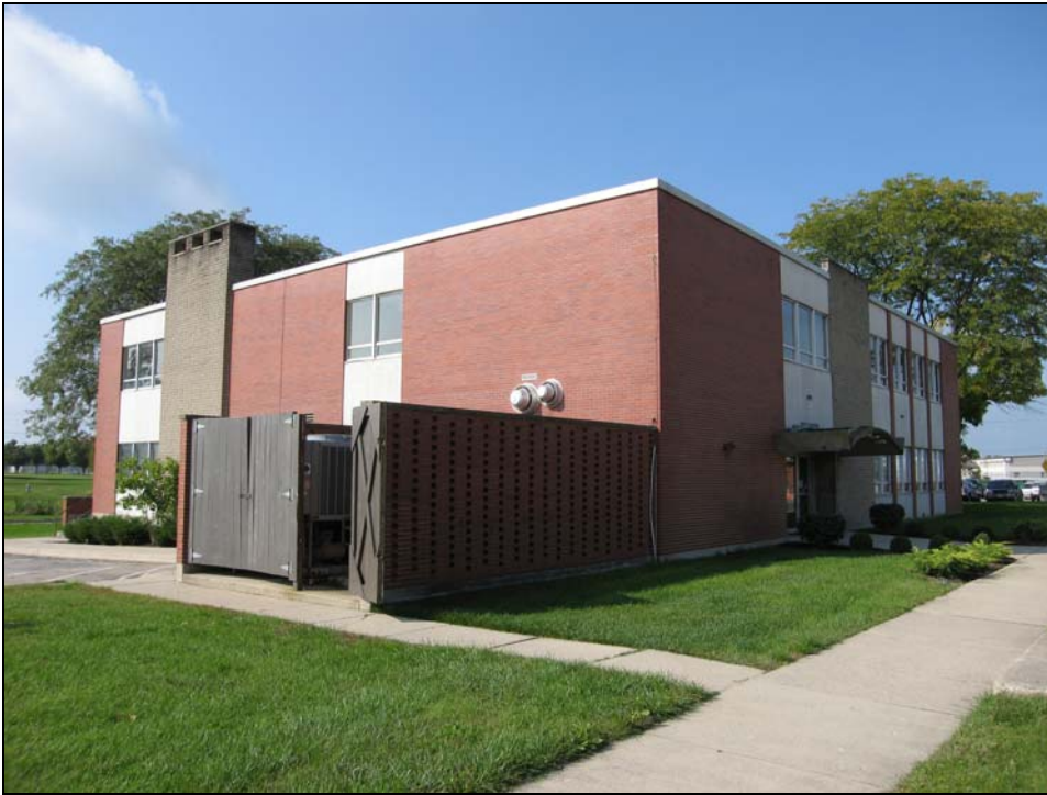
Figure 70. Building 31222, northeast corner, looking southwest
