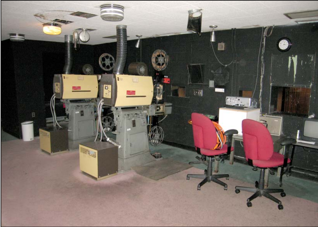
Figure 84. Building 31239, second-floor projection room, looking southwest
