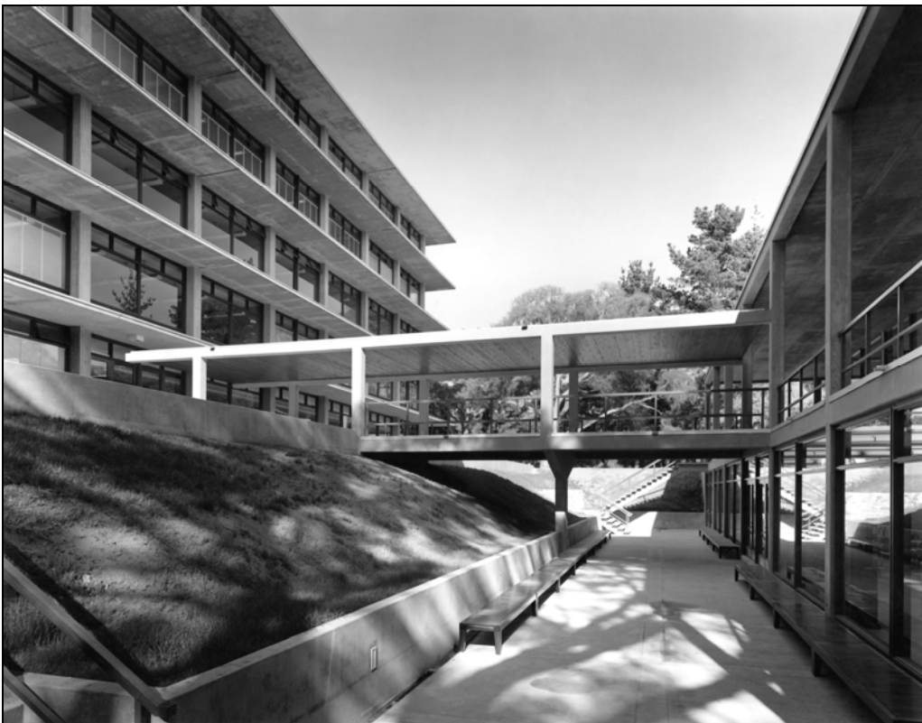
Figure 27. General Classroom and Office Building (built 1952–1954), Naval Postgraduate School, Monterey, California, designed by SOM
