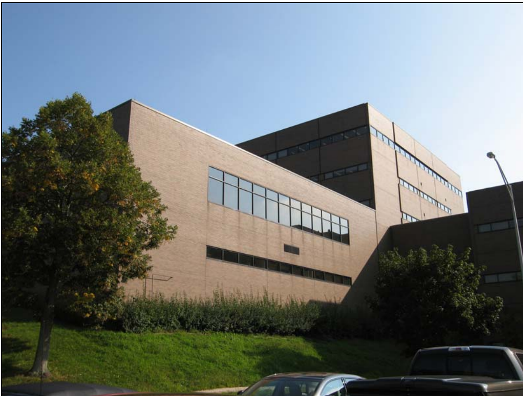
Figure 65. Building 20653, southwest corner, looking northeast
