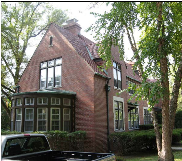
Figure 15. Brick Quarters Officer Housing Unit (built 1935–1936), Wright-Patterson Area A, designed by Albert Kahn and Louis Lott
