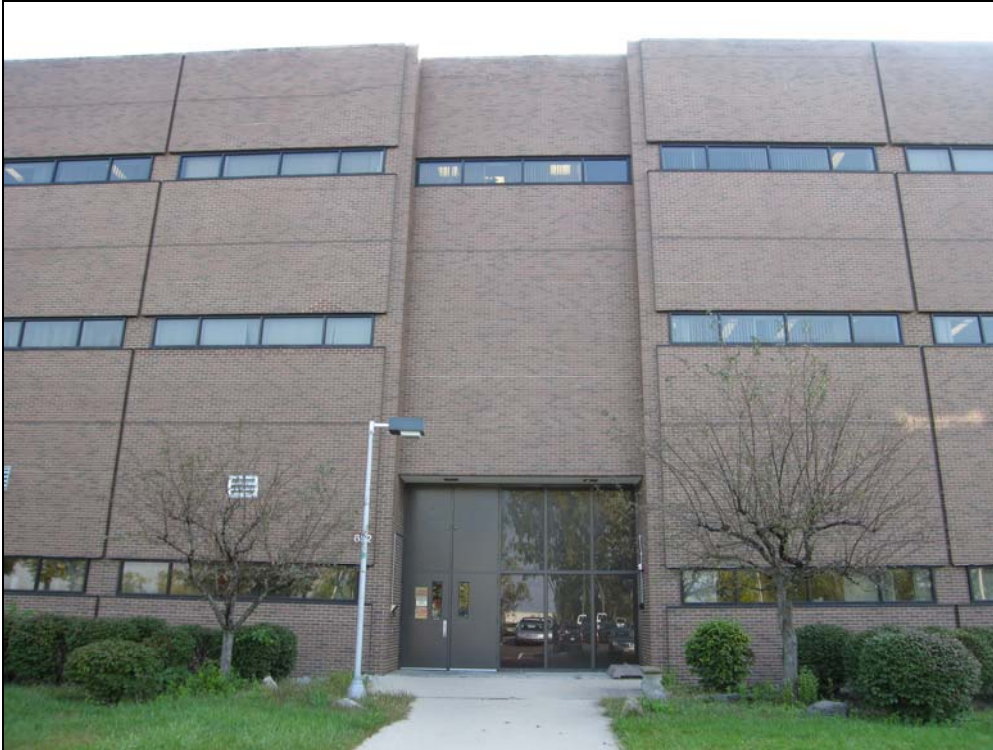
Figure 60. Building 20652, west wall, looking east
