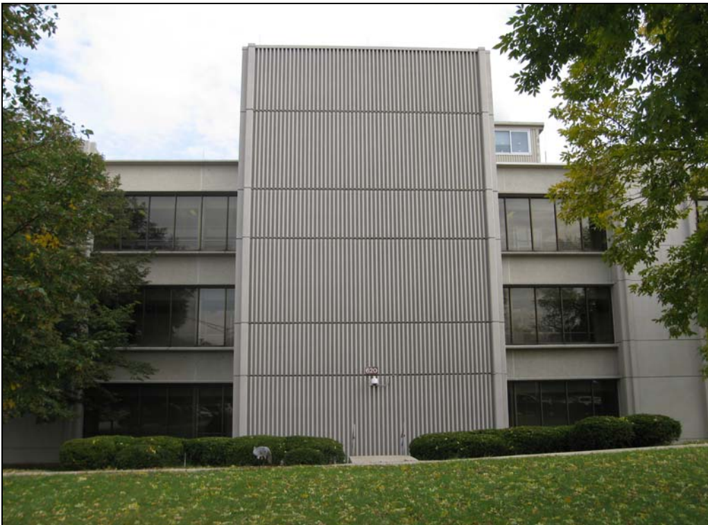
Figure 50. Building 20620, south wall, looking north, original 1966–1967 portion of building
