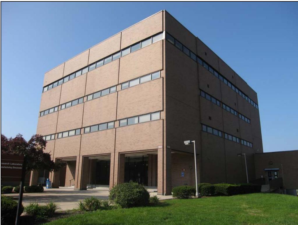
Figure 63. Building 20653, northeast corner, looking southwest
