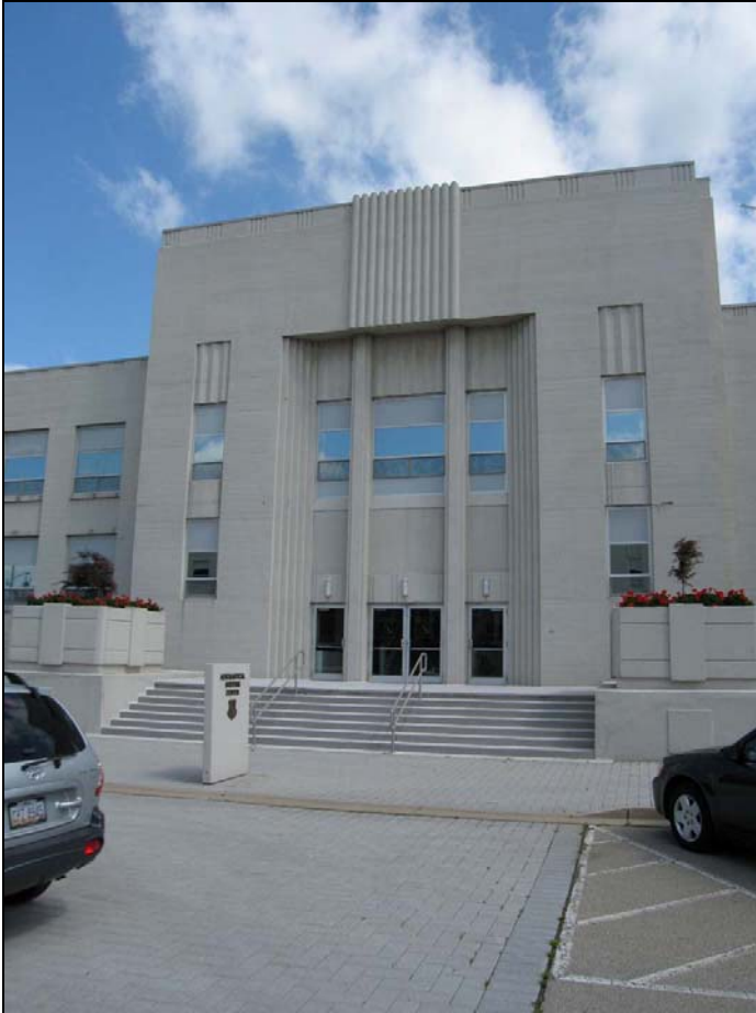
Figure 11. Building 20014 (built 1943), Wright-Patterson Area B, designed by Sverdrup & Parcel, Engineers, and J. Gordon Turnbull, view of entrance bay
