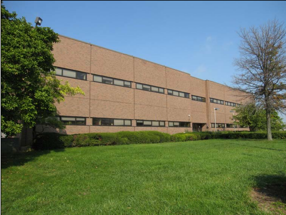
Figure 56. Building 20651, southeast corner, looking northwest
