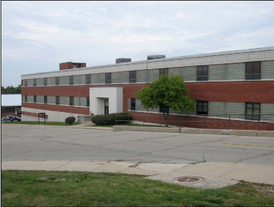
Figure 19. Building 20028, Aircraft Radio Laboratory (built 1942) at Wright-Patterson Area B
