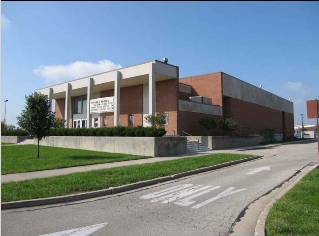
Figure 77. Building 31239, northeast corner, looking southwest
