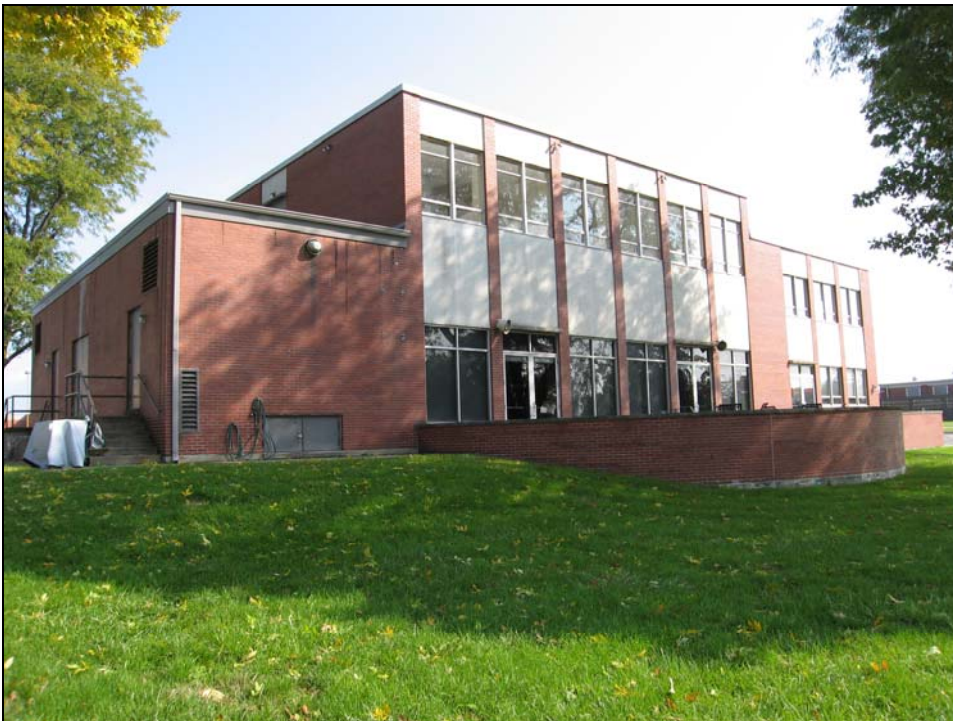
Figure 71. Building 31222, southwest corner, looking northeast
