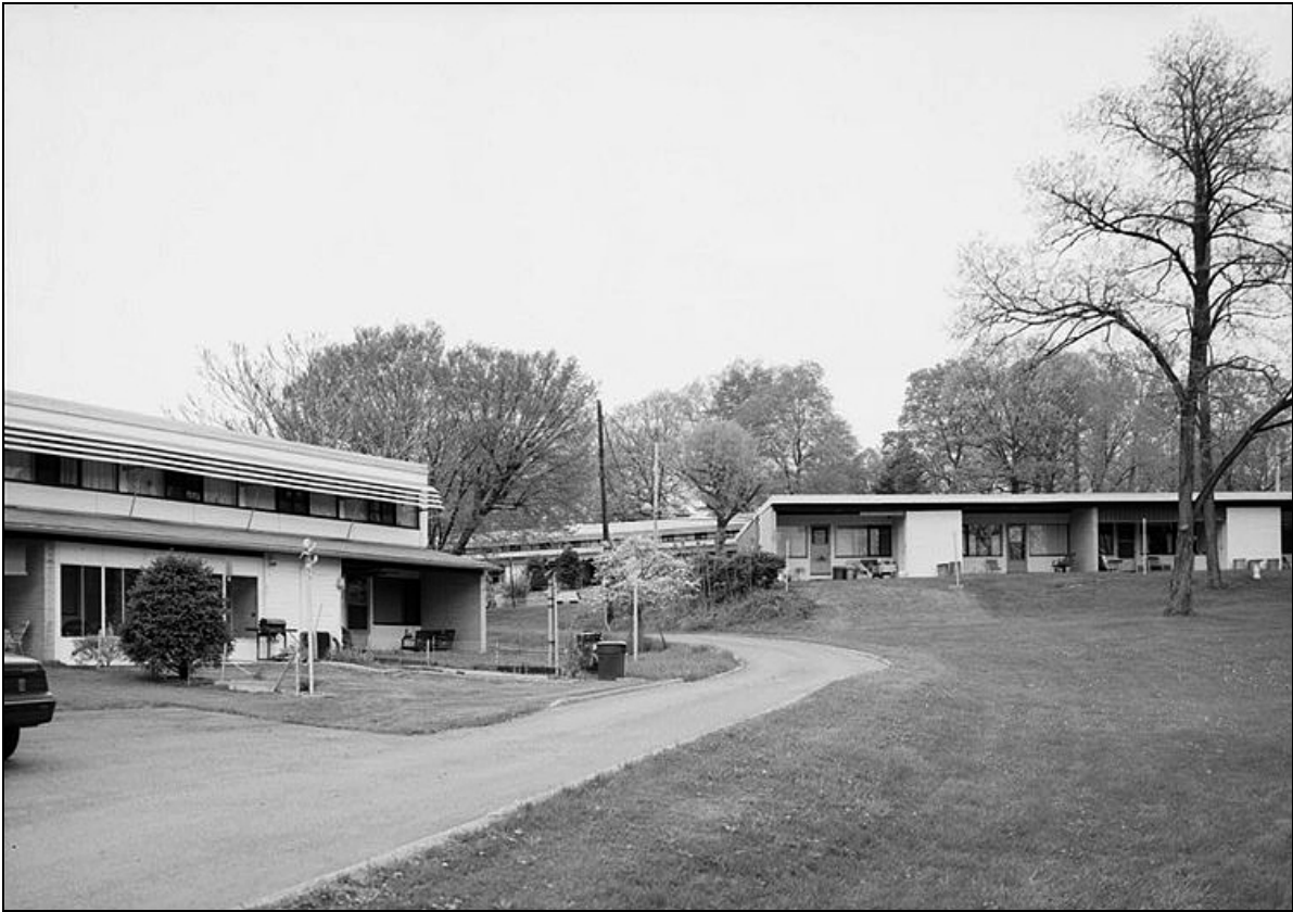
Figure 16. Aluminum City Terrace (built 1941), New Kensington, Pennsylvania, designed by Walter Gropius and Marcel Breuer
