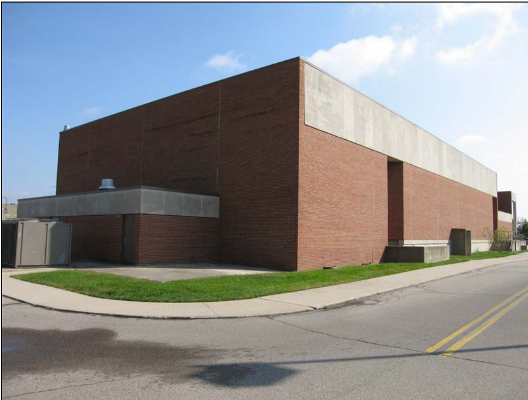
Figure 81. Building 31239, southwest corner, looking northeast
