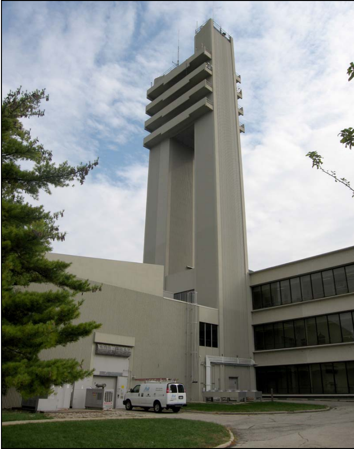
Figure 48. Building 20620, tower looking northeast, original 1966–1967 portion of building
