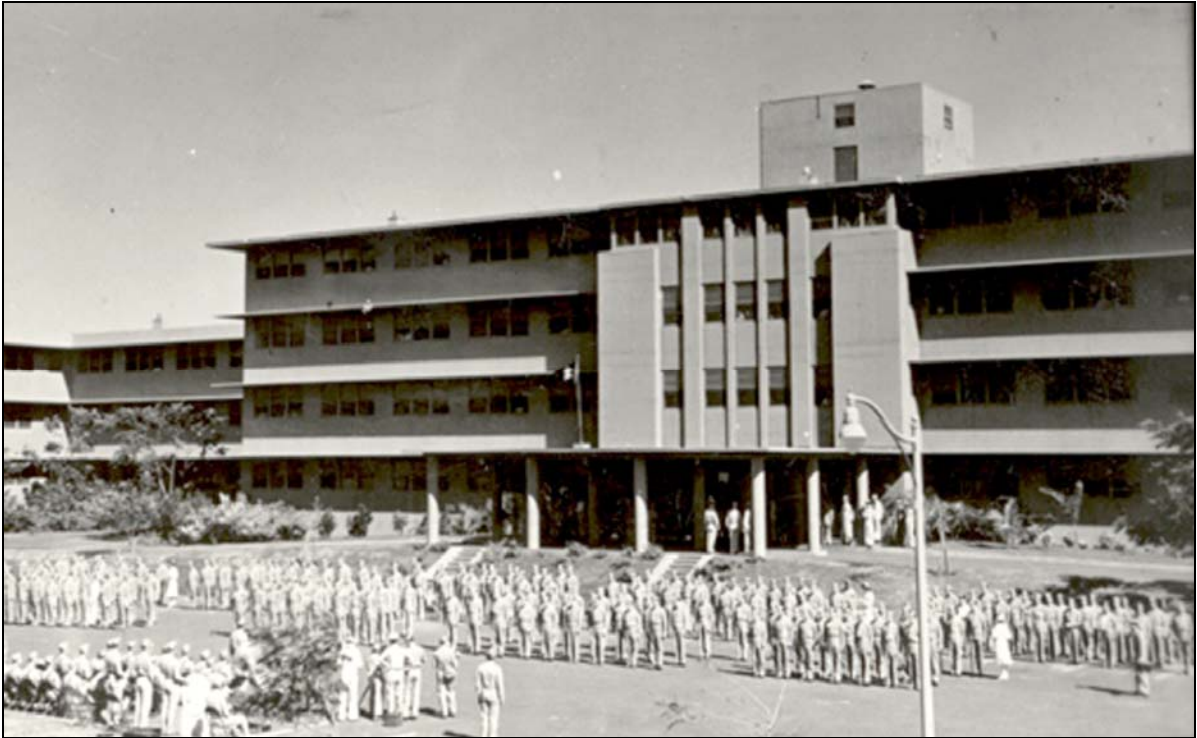
Figure 22. Aiea Naval Hospital (built 1942), Hawaii, designed by Charles W. Dickey Photo by the Honolulu Star-Bulletin , 27 October 1944, provided by the University of Hawaii Library
