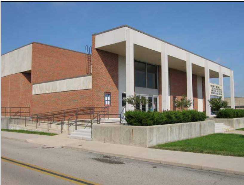
Figure 46. Building 31239, Base Theater (built 1966), Wright-Patterson Area A, designed by Daniel, Mann, Johnson & Mendenhall
