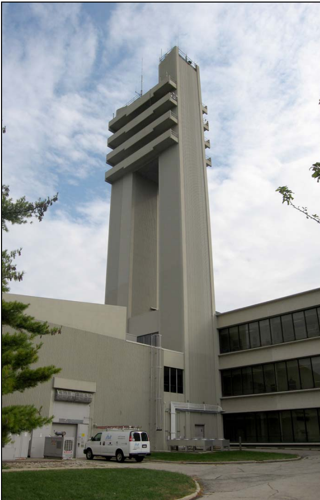
Figure 43. Building 20620 (built 1966–1967), tower, Wright-Patterson Area B, designed by Dalton & Dalton
