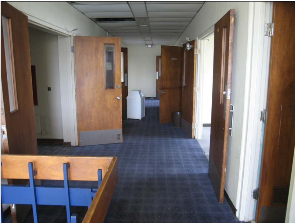
Figure 75. Building 31222, second-floor corridor, looking west
