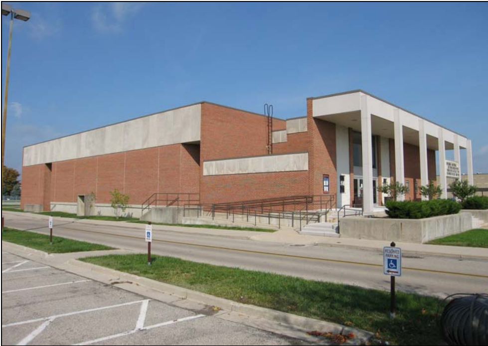
Figure 78. Building 31239, southeast corner, looking northwest
