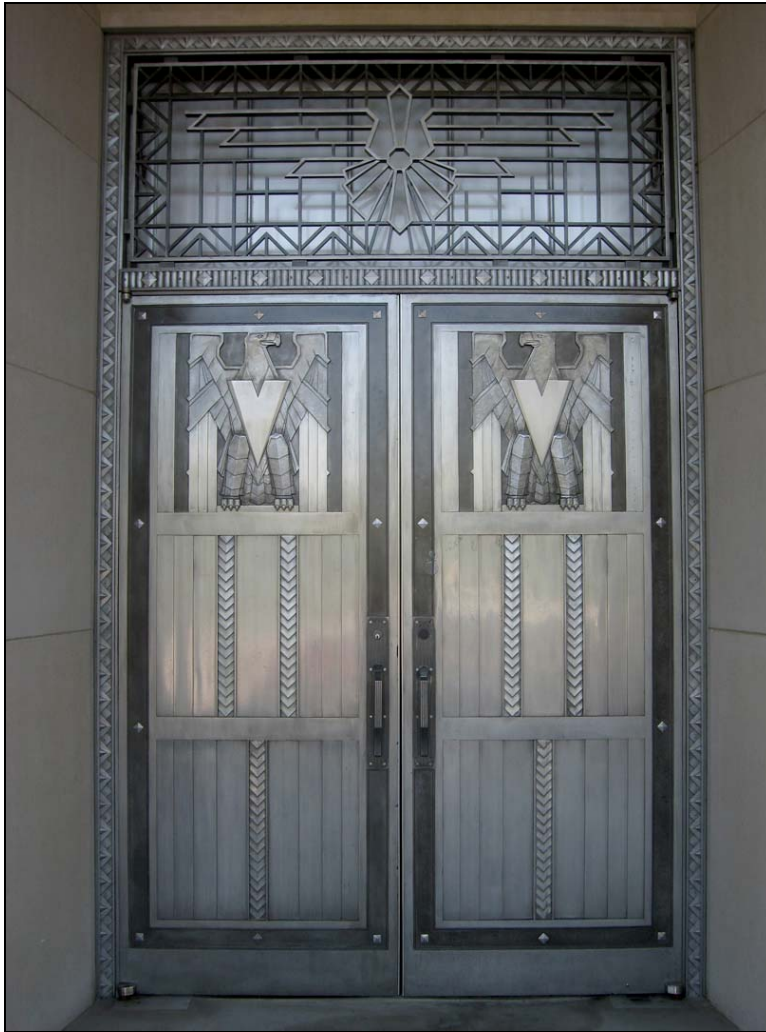
Figure 9. Building 20012, front entrance double doors
