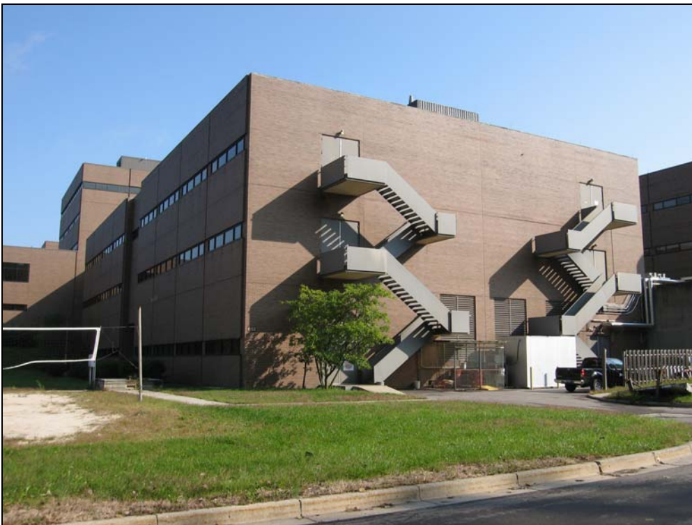
Figure 59. Building 20652, southwest corner, looking northeast
