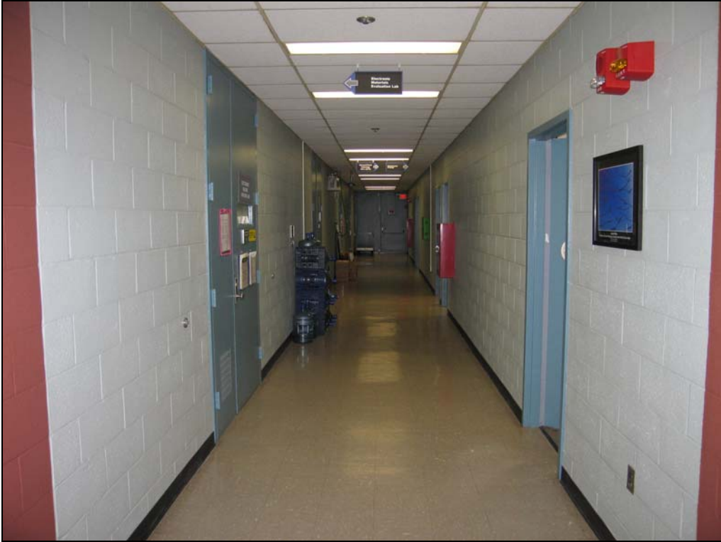
Figure 62. Building 20652, second-floor corridor, looking west
