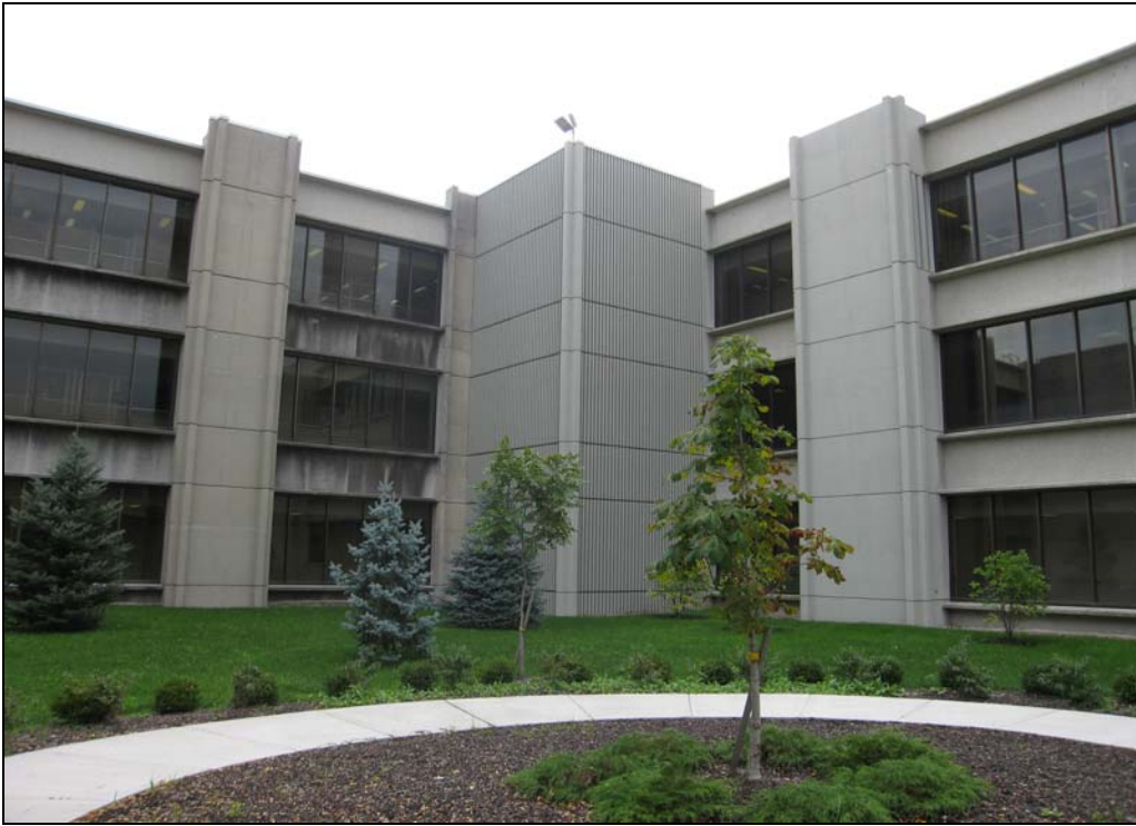
Figure 49. Building 20620, courtyard looking southeast, original 1966–1967 portion of building
