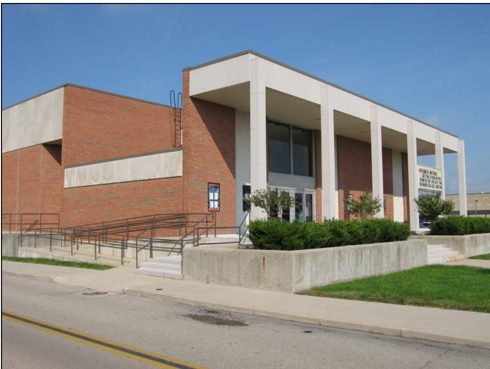
Figure 79. Building 31239, detail of portico, looking northwest
