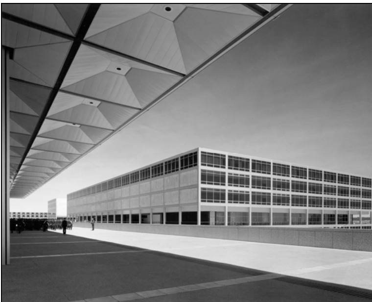
Figure 34. Fairchild Hall (built 1956–1962), U.S. Air Force Academy, Colorado, designed by SOM Photo by Hedrich Blessing, ca. 1962
