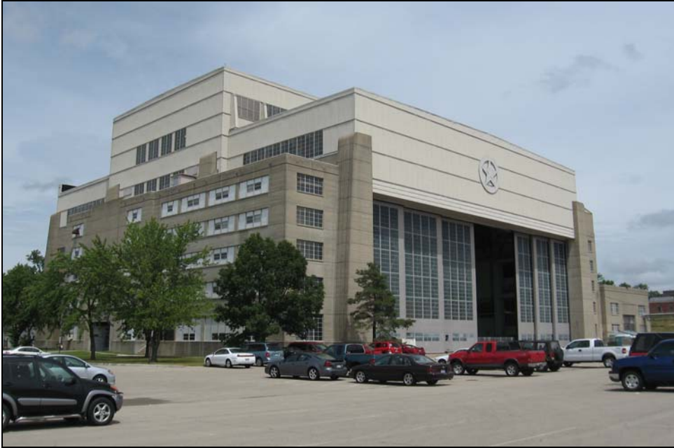
Figure 13. Building 20065 (built 1944), Wright-Patterson Area B, designed by Hazelet & Erdal, Engineers
