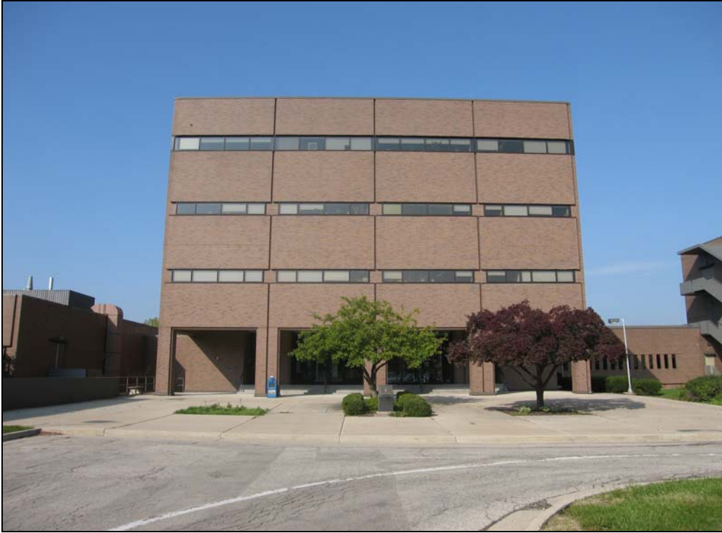
Figure 64. Building 20653, east wall, looking west
