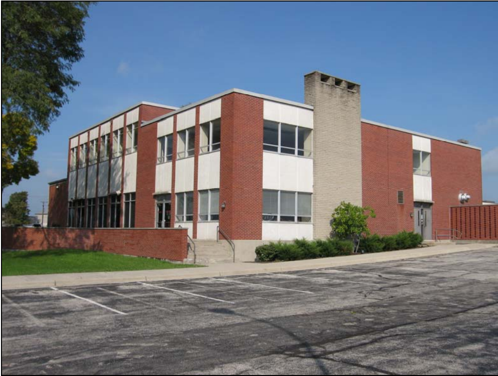
Figure 69. Building 31222, southeast corner, looking northwest
