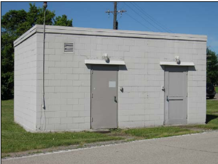
Figure 1. Building 34040, Former Water Treatment Facility (built 1960), Wright-Patterson Area A
