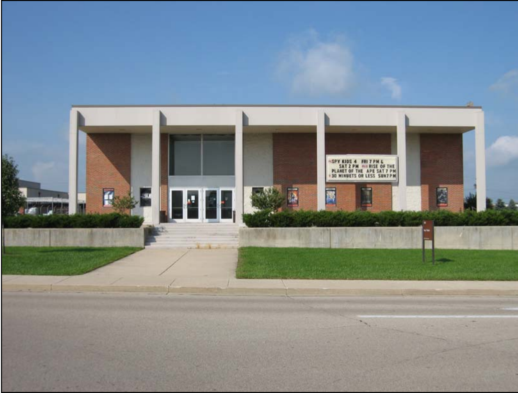
Figure 80. Building 31239, east wall and portico, looking west
