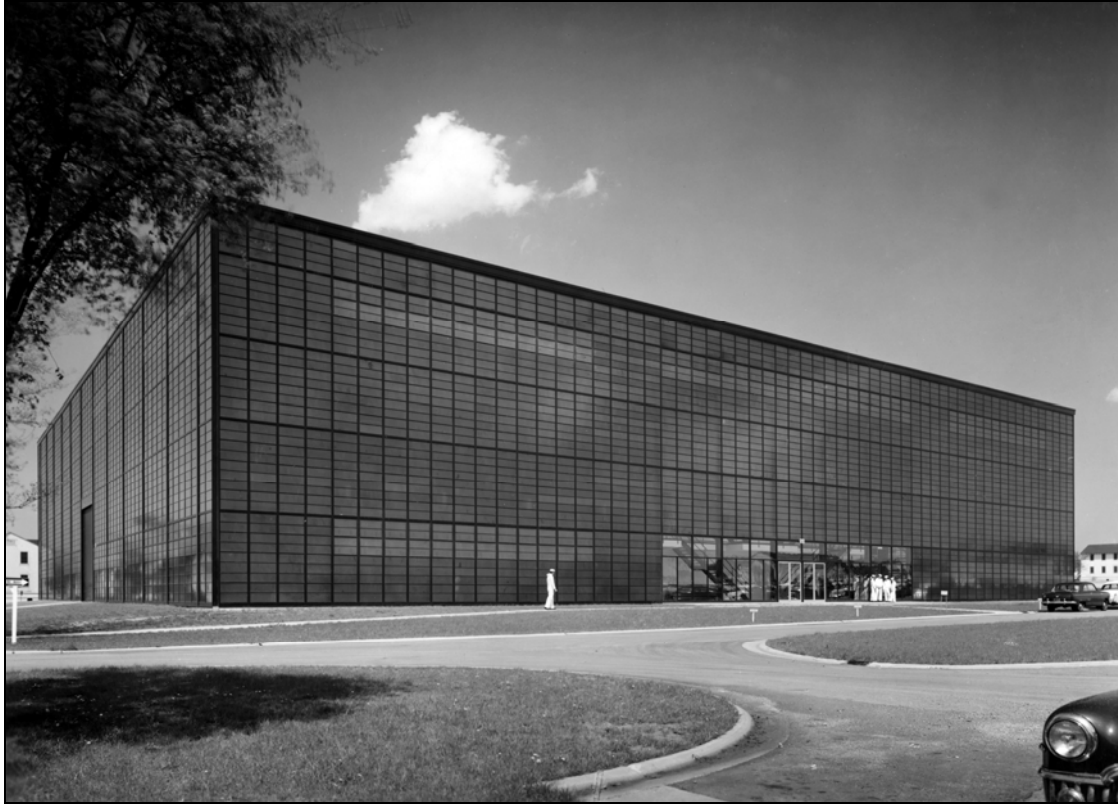
Figure 28. Building 521 (built 1952–1954, demolished 2010), Naval Station Great Lakes, Illinois, designed by SOM Photo by Hedrich Blessing, 1954
