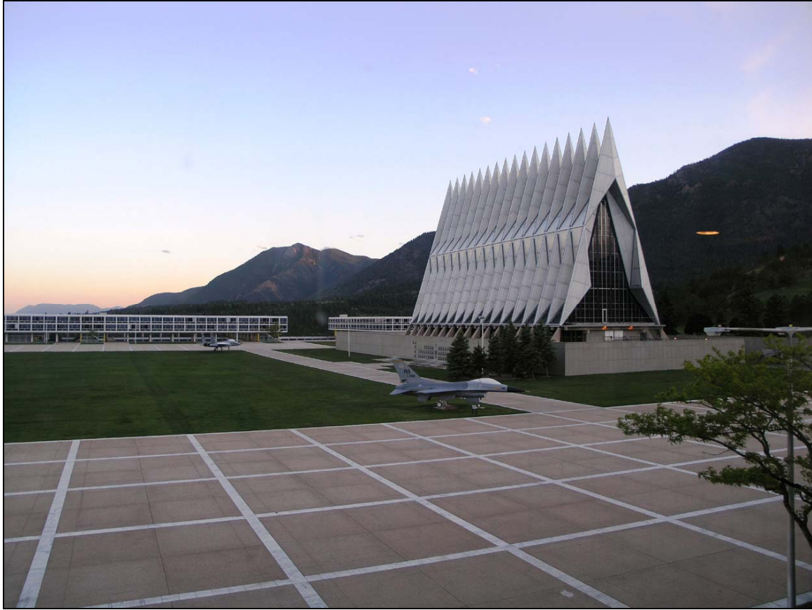
Figure 31. View of the U.S. Air Force Academy, Colorado, showing the Chapel (built 1956–1962), designed by SOM Photo by Skidmore, Owings & Merrill, ca. 2005
