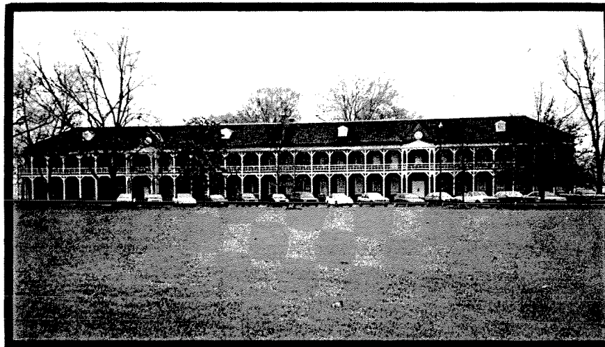
Figure III-109. 1883 Wood-frame barracks (Building 22208, Ft. Huachuca, Arizona), above . 1893 Multiple-company barracks (Building 111, Ft. Bliss, Texas), middle . 1891 Barracks with simplified Queen Anne and Stick style detailing (Building 58, Ft. McPherson, Georgia), below
