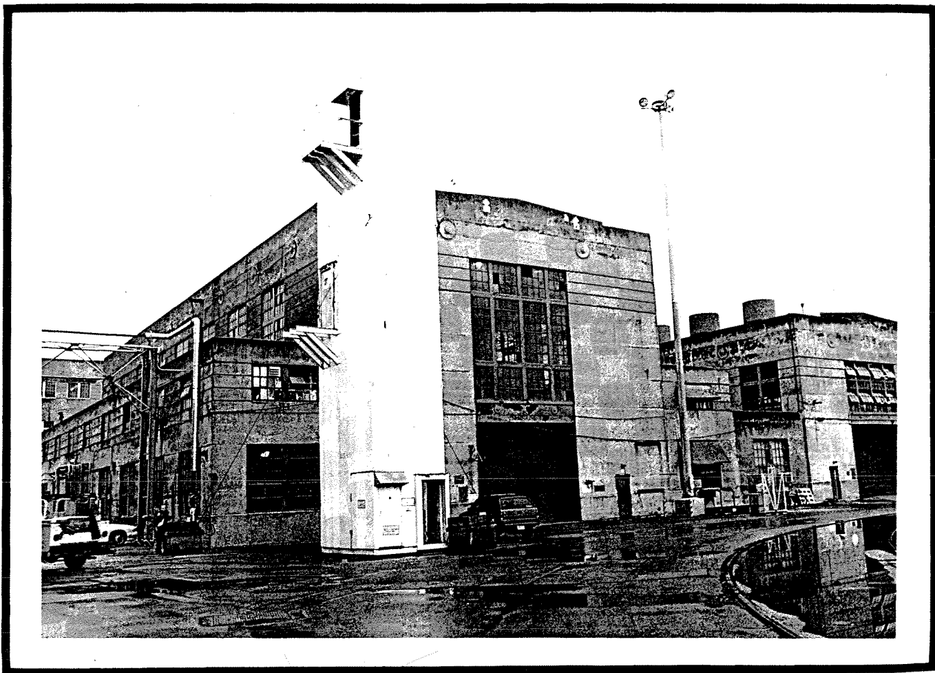
Figure III-61. 1938-1939 Forge shop (Building 452, Naval Shipyard Puget Sound, Bremerton, Washington), above . 1937 Pipe and copper shops (Building 56, Naval Base Charleston, South Carolina), below . (Courtesy U.S. Navy)
