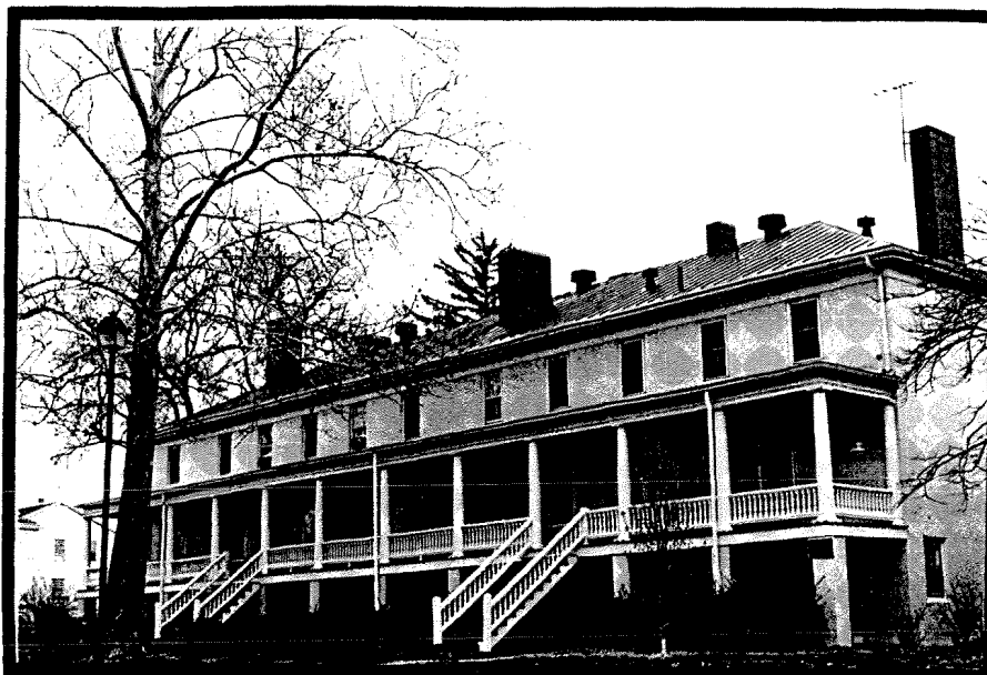
Figure III-129. Officers housing at Ft. Monroe, Virginia (no longer extant), above , and 1823 Officers quarters (Buildings 17 and 18, Ft. Monroe, Virginia), middle . (From National Archives, Record Group 77, Fortifications Files, Ft. Monroe, Virginia.) Ca. 1832 Officer housing (Building 19, Ft. Leavenworth, Kansas), below
