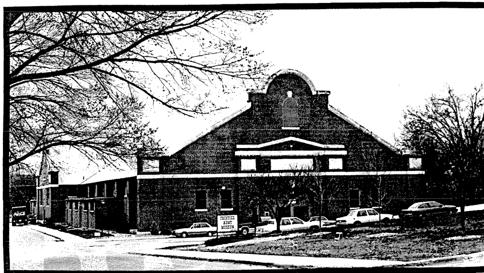
Figure III-31. 1907-1908 Cavalry Riding Halls, Quartermaster standardized plan no. 97-A: F.E. Warren AFB [formerly Ft. D.A. Russell], Wyoming (Building 314), above , Ft. Riley, Kansas (Building 127), middle , and Ft. Leavenworth, Kansas, (Building 302), below .
