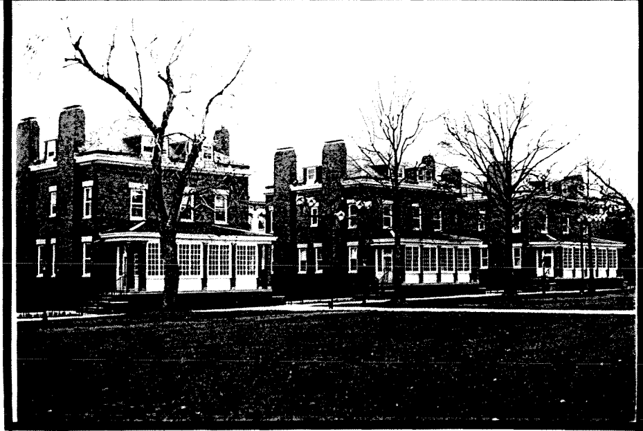
Figure III-152. 1801 Commandant's house, mansard roof added 1891 (U.S. Marine Corps Barracks, Washington, D.C.), above . (Courtesy U.S. Marine Corps) Officers housing constructed between 1903 and 1907 (U.S. Marine Corps Barracks, Washington, D.C.), below
