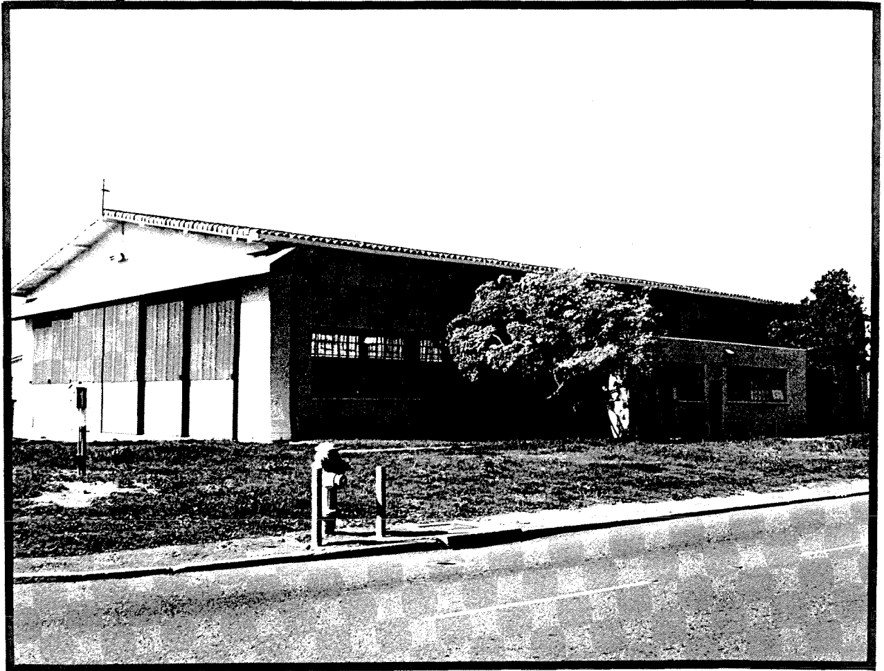
Figure III-160. 1918 Hangar, Albert Kahn, architect (Building 781, Langley AFB, Virginia), above . 1918 Hangar, Albert Kahn, architect (Building 502, Naval Air Station North Island [formerly Rockwell Field], San Diego, California), below
