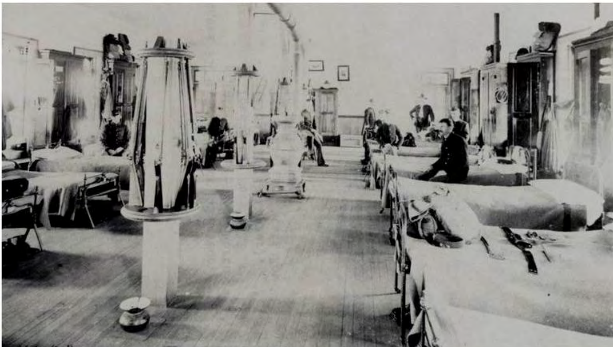
Figure 12: Interior photograph of Building 56 at Fort MacPherson, ca. 1900
