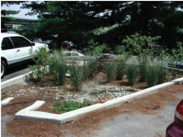
Figure 29: Bioswale at Navy Yard
