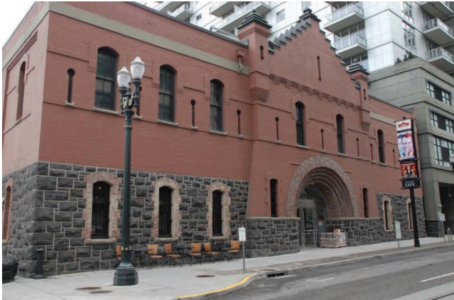
Figure 10: The Gerding Theater at the Armory (Annex) facade
