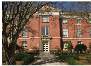
Charleston Navy Yard, Building 7
