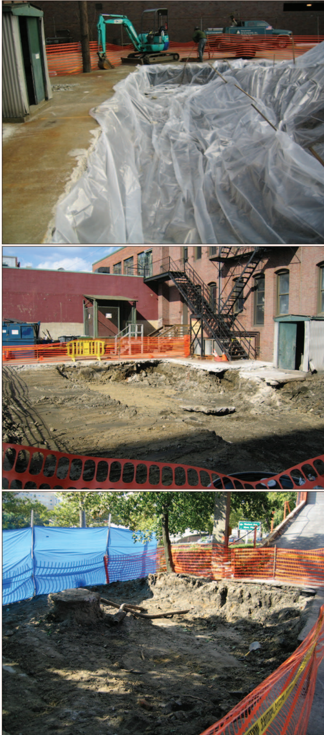
Figure 26: Soil remediation for 46 Blackstone South at different stages
