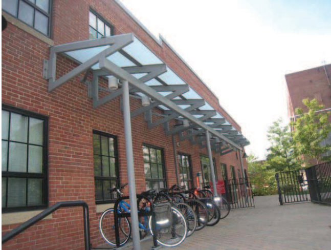
Figure 47: Covered bicycle parking near the front entrance
