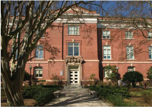
Figure 7: Charleston Navy Yard, Building 7
