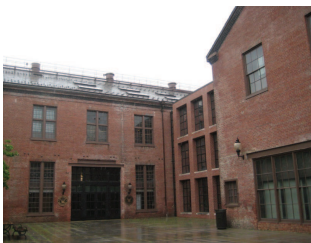
Washington Navy Yard, Building 33
