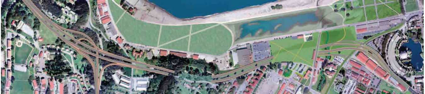
Figure 24: Aerial view of Doyle Drive
