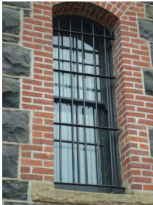
Figure 27: Exterior view of historic double hung, wood window
