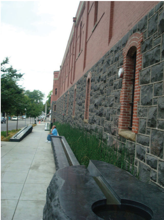
Figure 39: Silver Park, formerly the location of a sidewalk and parking spaces, incorporates native vegetation, a small water feature with recirculating stormwater treatment
