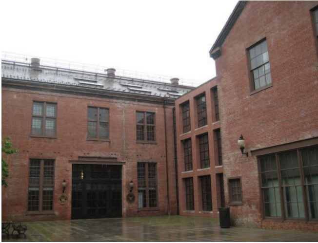
Figure 4: Building 33 Courtyard View
