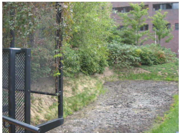
Figure 35: Bioswale surrounded by native trees and bushes including pin oak, river birch and honey locust. Waterline aligns gravel edge
