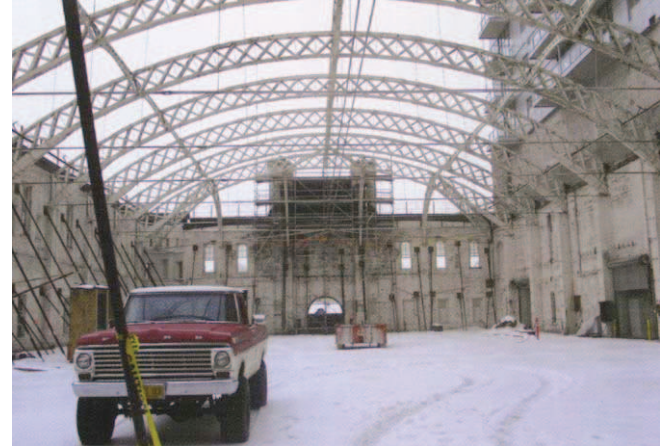
Figure 41: Armory during construction without roof
