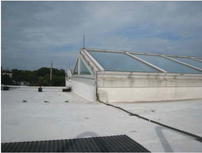
Figure 43: White thermo plastic olefin roof
