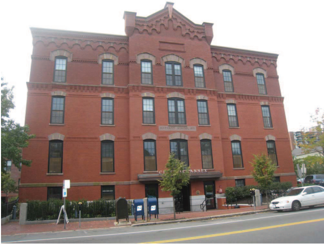
Figure 11: Cambridge City Hall Annex facade
