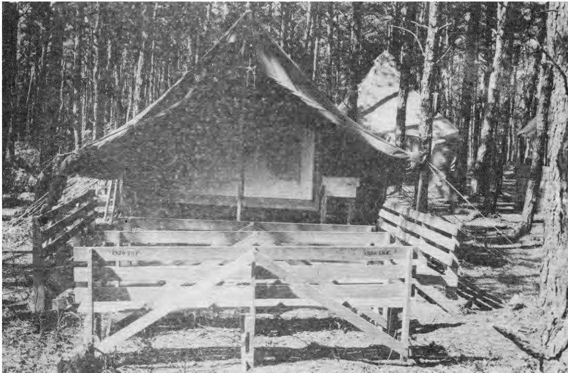
Figure 259. Improvised outdoor classrooms (Becker, 1946, p 33).
