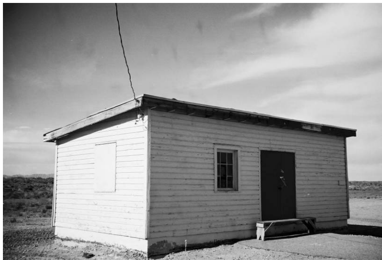
Figure 322. WWII range target storage building 9898, Fort Bliss, TX, November 2005.
