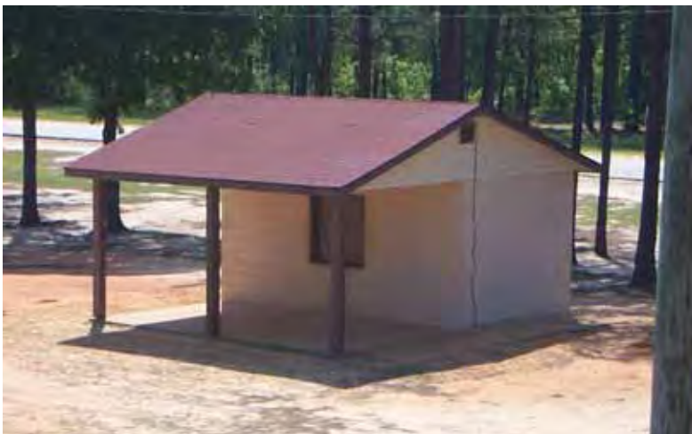
Figure 337. Range ammunition storage building, Fort Bragg, 17 May 2006.
