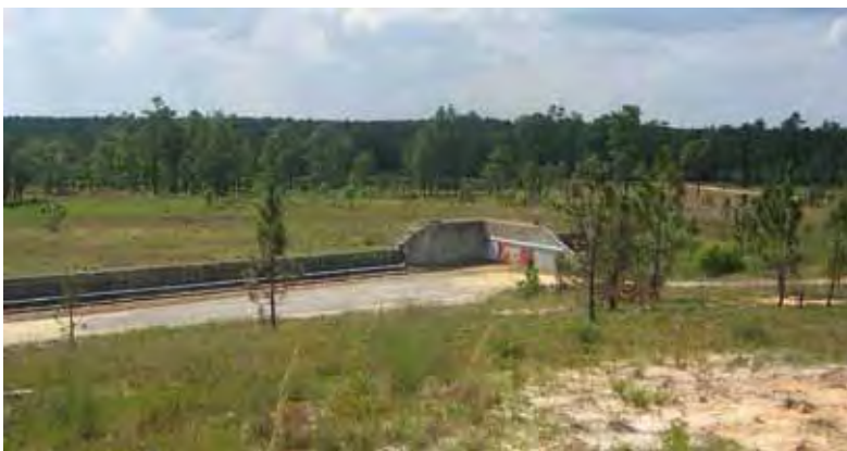
Figure 302. Target storage and repair building at the end of the target track protected by an embankment, Fort Bragg, 17 May 2006.
