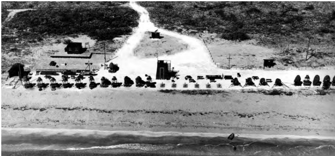
Figure 108. Beach firing range at NAS Fort Lauderdale, FL, 28 February 1944 (NARA College Park, RG 80-G, box 1513, photo 388275).
