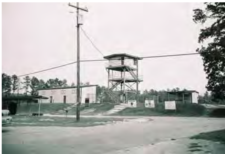
Figure 347. 1995 Range 10 observation tower and grandstand, Fort Jackson, July 2003.
