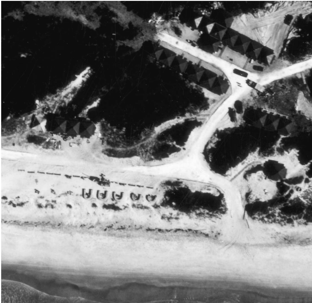
Figure 109. Aerial of machine gun range at MCAS Cherry Point, NC, 9 August 1943 (NARA College Park, RG 80-G, box 1495, photo 384685).
