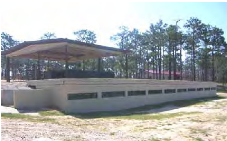
Figure 348. Range bleachers, Fort Bragg, 17 May 2006.
