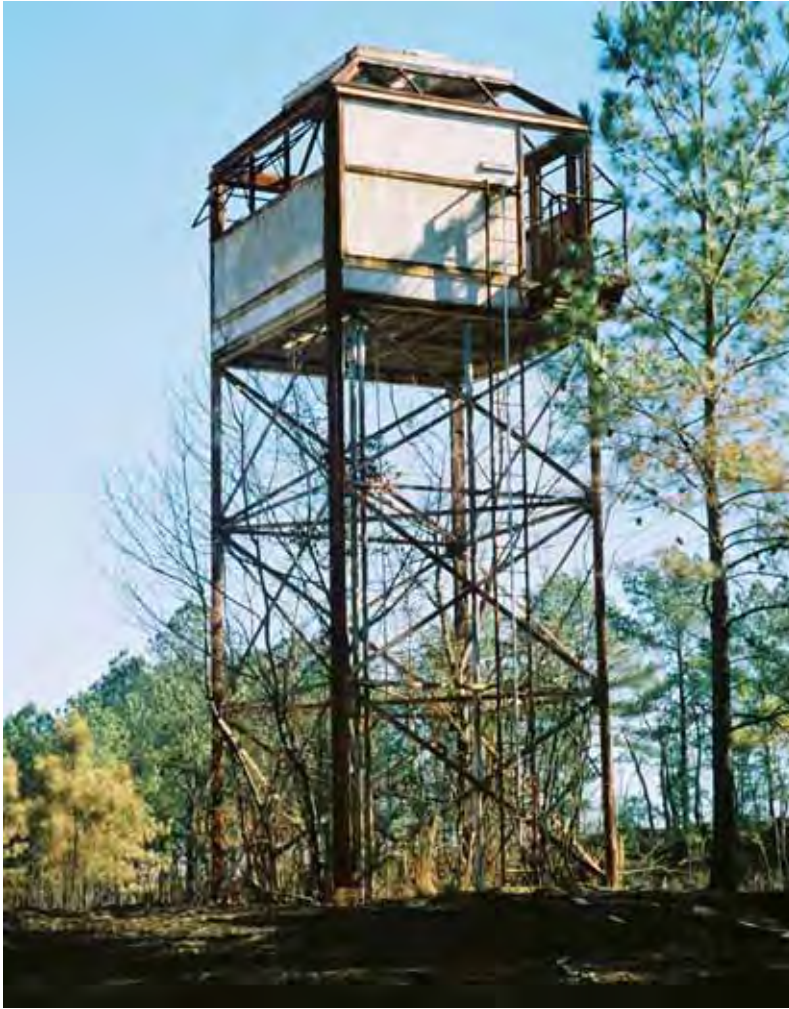
Figure 313. 1966 observation tower near Old Range #19, Fort Gordon, GA, January 2004.
