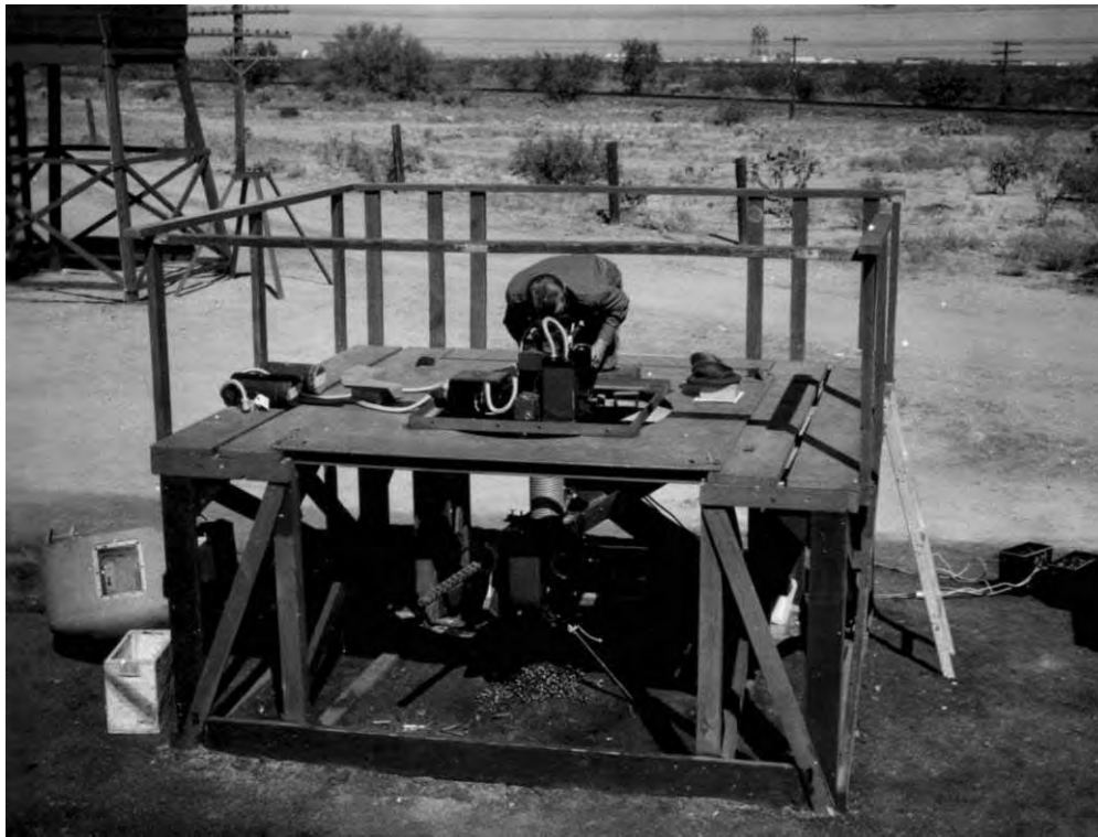
Figure 21. Installation of consolidated gun turret on machine gun range at Davis-Monthan Field (Tucson), AZ, 2 November 1942 (NARA College Park, RG 342-FH, box 2202, photo 4A-17356).
