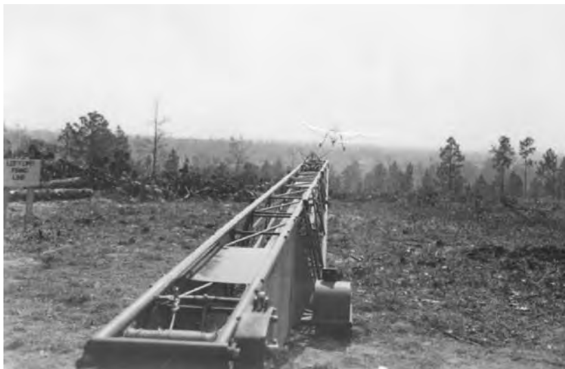
Figure 118. Radio-controlled airplane target OQ-2A taking off from catapult at the AA Range at Fort Jackson, SC, 1 November 1943 (NARA College Park, RG 111-SC WWII, box 415, photo SC246692).
