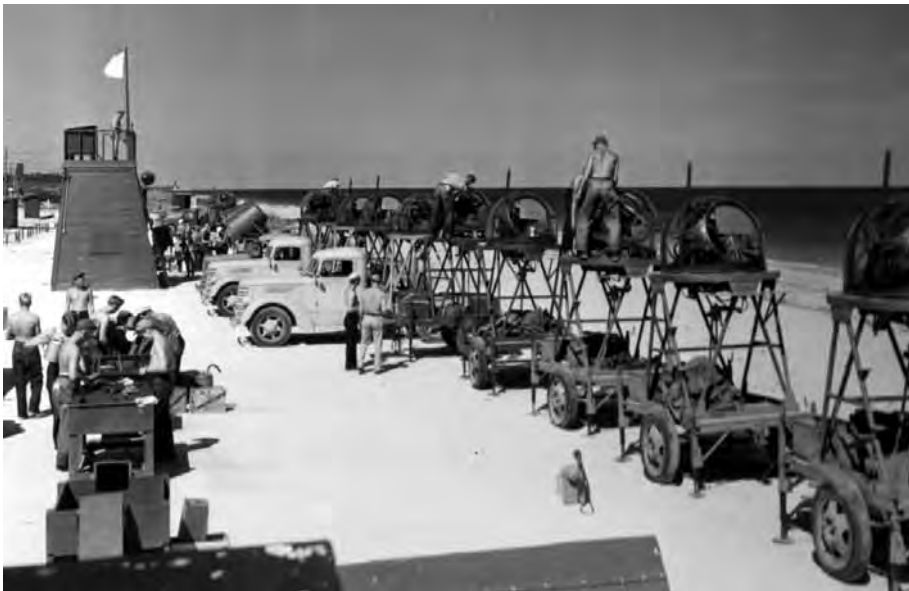
Figure 111. Beach firing range at NAS Fort Lauderdale, FL, 28 February 1944 (NARA College Park, RG 80-G, box 1513, photo 388274).
