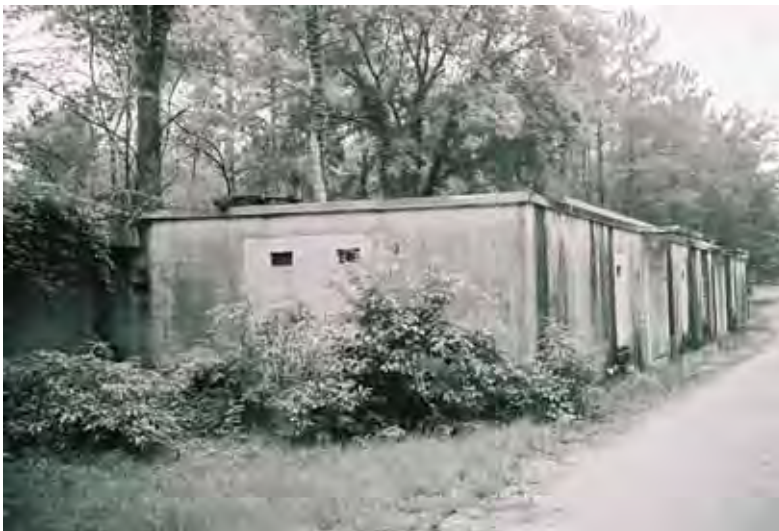
Figure 342. Remains of WWII known distance range target butt, latrine, and target storage, Fort Jackson (SCARNG), June 2004.
