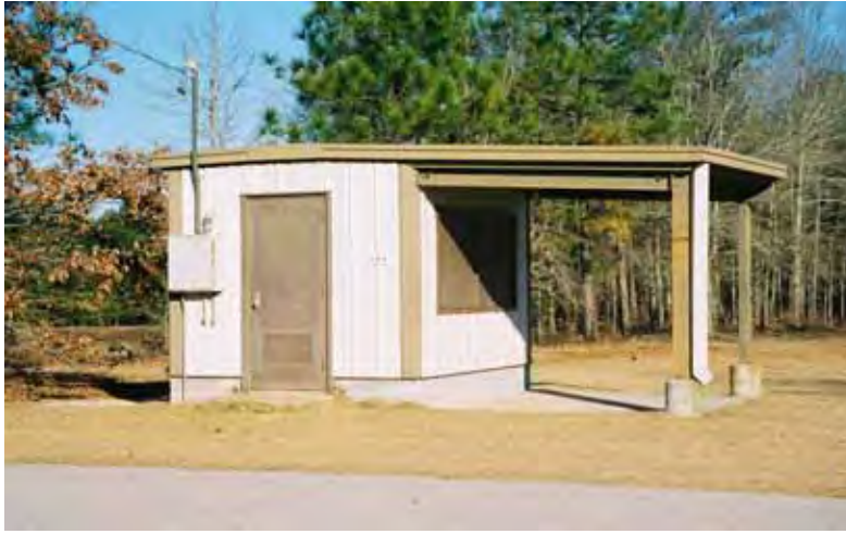
Figure 335. 1987 Bldg 485 range storage, Fort Gordon, GA, January 2004.
