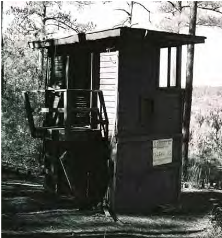
Figure 311. Remains of 1950s observation tower on Combat II Range, Fort Jackson, June 2004.
