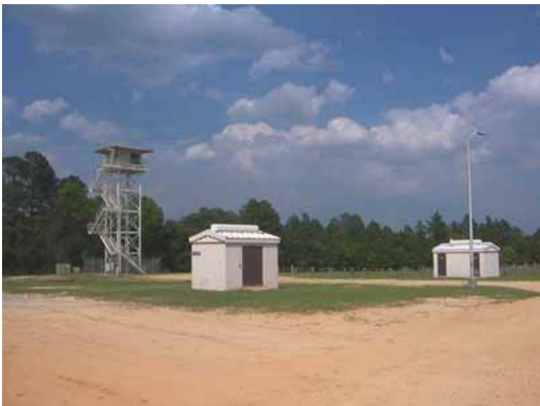
Figure 317. Control tower and range buildings, Fort Bragg, 17 May 2006.
