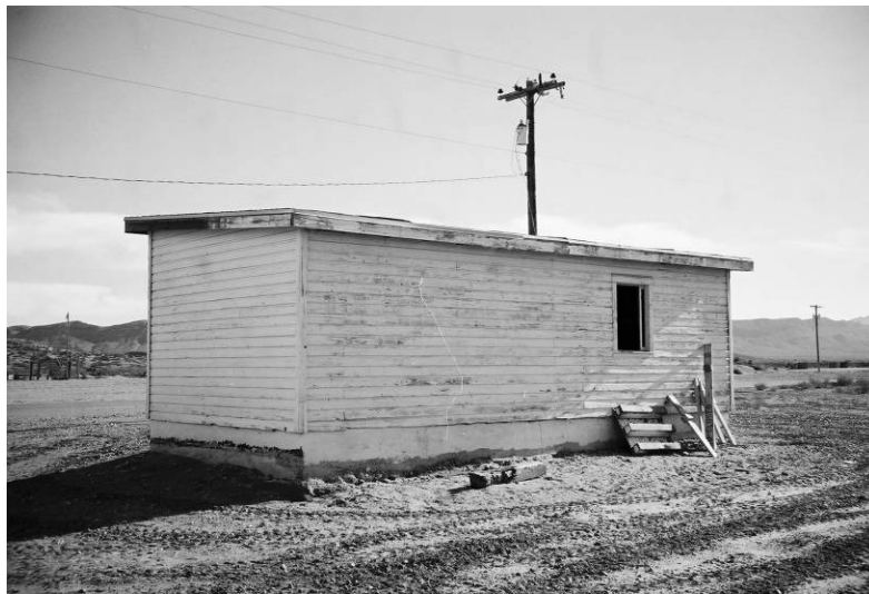
Figure 321. WWII range target storage building 9898, Fort Bliss, TX, November 2005.
