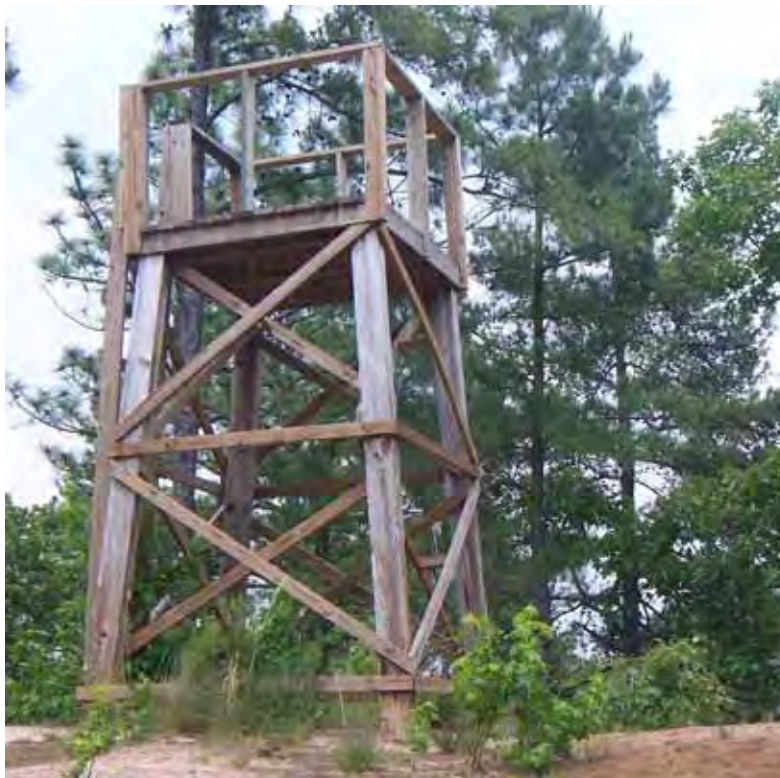
Figure 312. observation tower, Fort Bragg, 17 May 2006.
