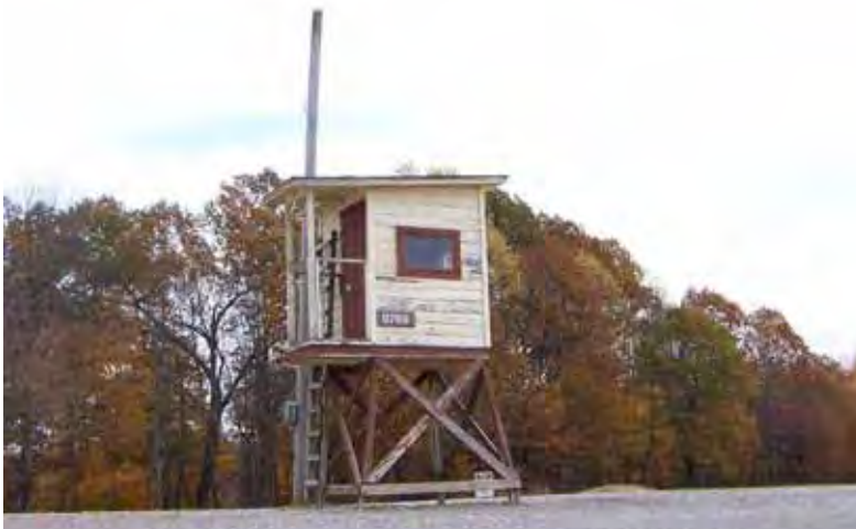
Figure 307. WWII observation tower Bldg 9789, Fort Knox, KY, November 2005.
