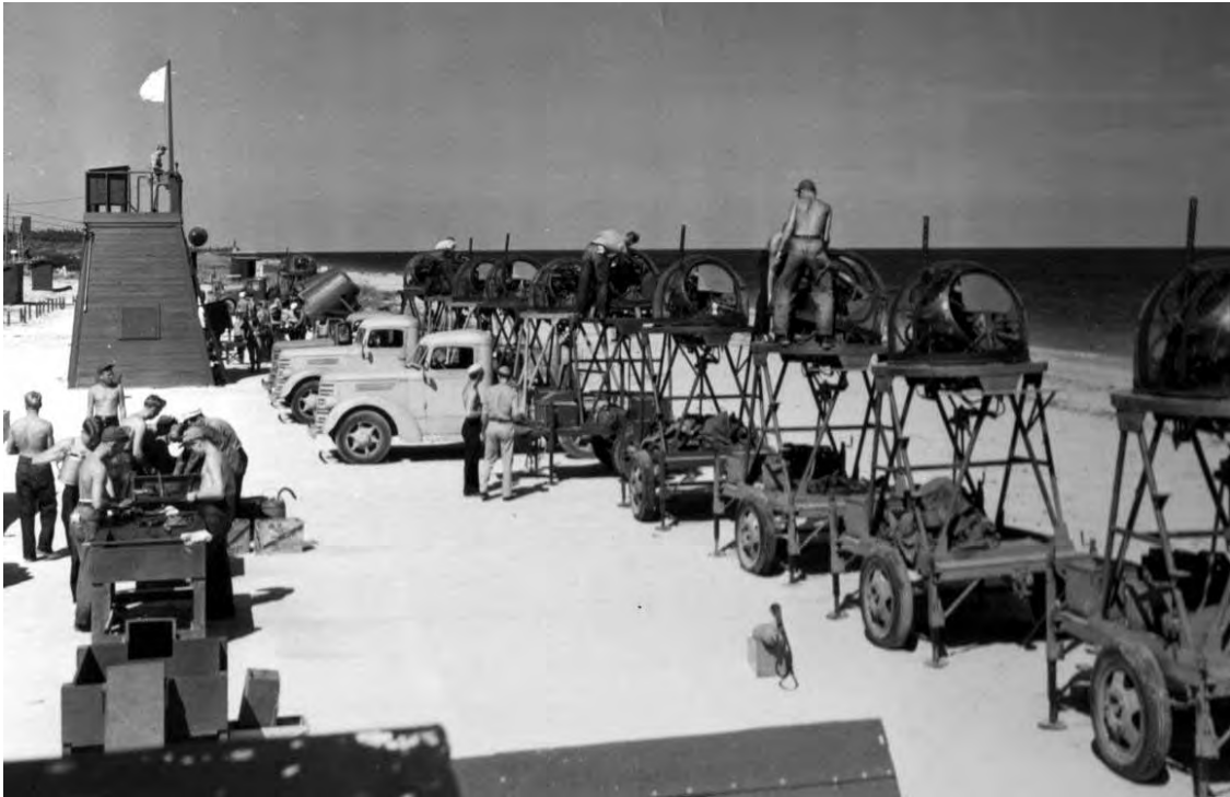
Figure 23. Beach firing range at NAS Fort Lauderdale, FL, 28 February 1944 (NARA College Park, RG 80-G, box 1513, photo 388274).
