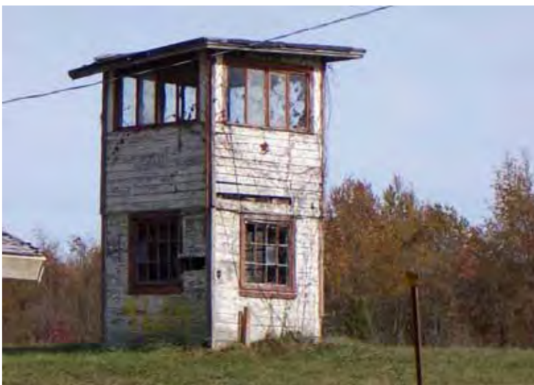
Figure 308. Remains of WWII observation tower Bldg 9606, Fort Knox, KY, November 2005.
