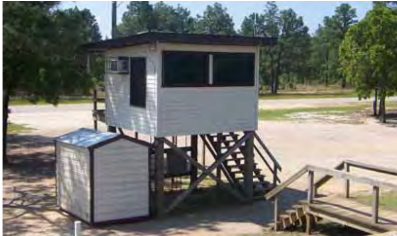
Figure 320. observation tower, Fort Bragg, 17 May 2006.
