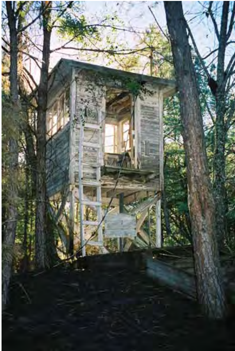
Figure 304. remains of WWII observation tower Bldg R122, Fort Gordon, GA, January 2004.
