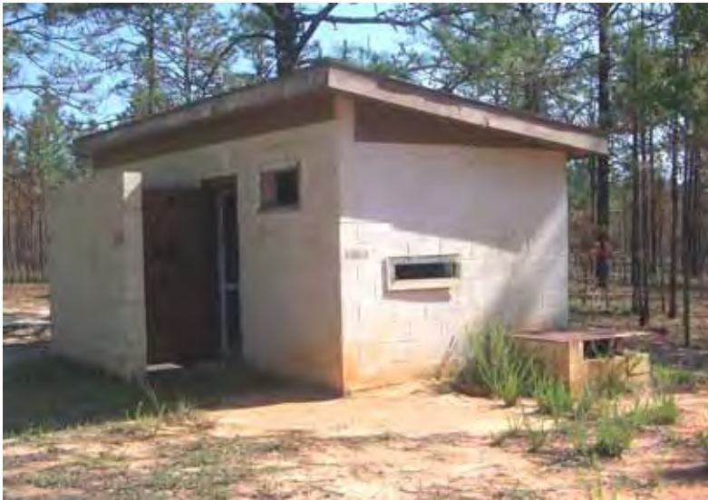
Figure 343. Range latrine, Fort Bragg, 17 May 2006.
