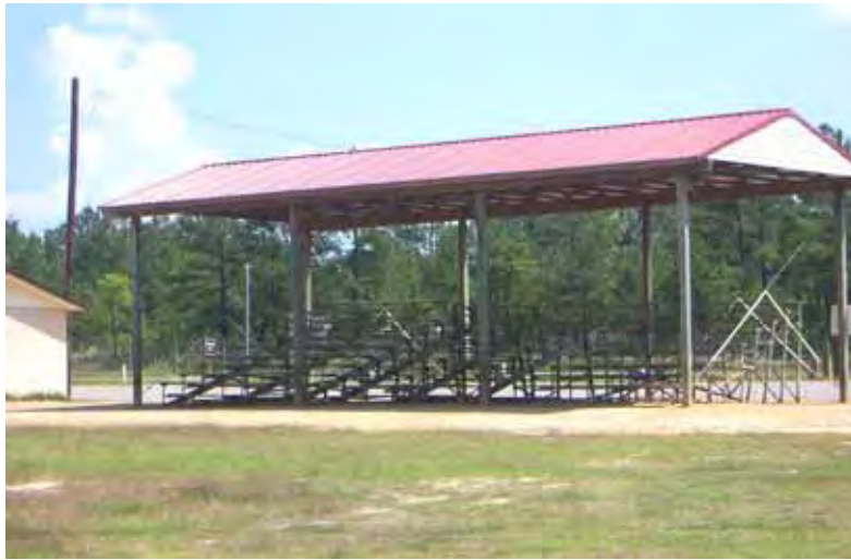
Figure 346. Range bleachers, Fort Bragg, 17 May 2006.
