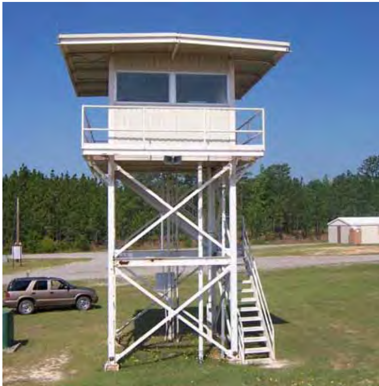
Figure 318. observation tower, Fort Bragg, 17 May 2006.
