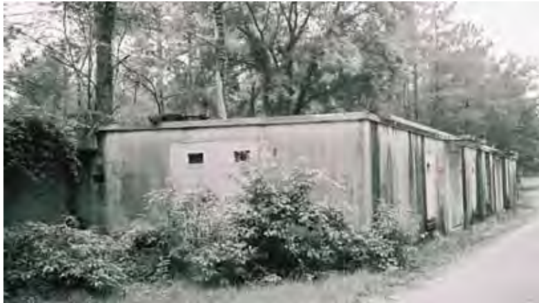
Figure 323. Remains of WWII known distance range target butt, latrine, and target storage, Fort Jackson (SCARNG), June 2004.
