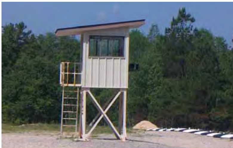
Figure 319. observation tower, Fort Bragg, 17 May 2006.
