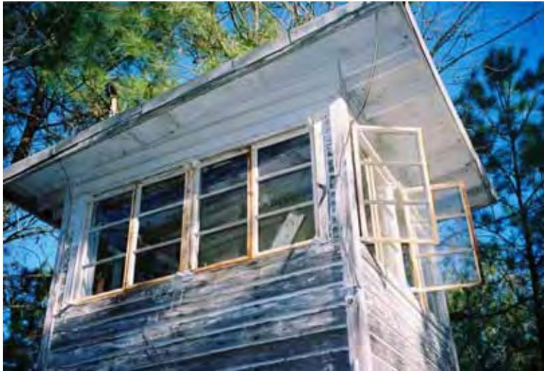
Figure 306. remains of WWII observation tower Bldg R122, Fort Gordon, GA, January 2004.
