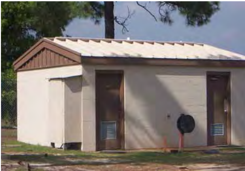
Figure 344. Range latrine, Fort Bragg, 17 May 2006.
