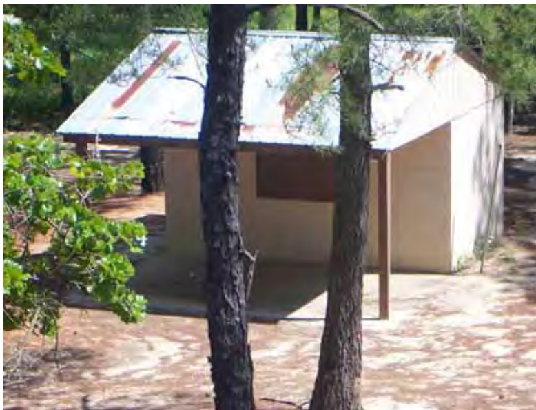
Figure 336. Range ammunition storage building, Fort Bragg, 17 May 2006.
