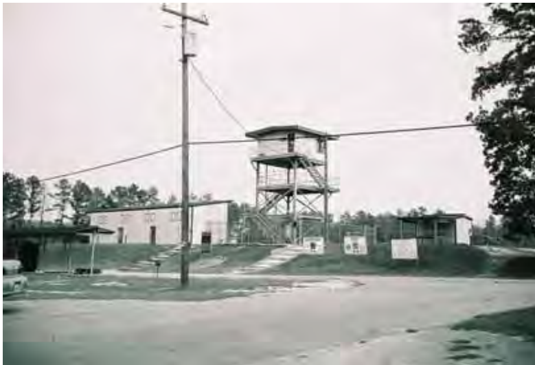
Figure 316. 1995 Range 10 observation tower and grandstand, Fort Jackson, SC, July 2003.
