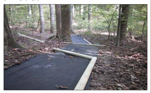
(Above: The objective of the project at USMC Base Quantico was to install at least 200ft. of erosion mitigation materials on the most eroded part of Hill Trail, which contains an archaeological site. The site of the project can only be reached on foot and the materials had to be carried over 600 meters of trail, crossing two streams and three fallen trees. Despite the difficulties, the project was a complete success.)
