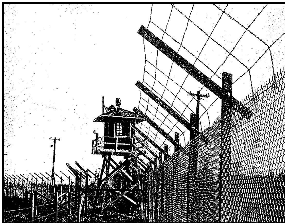
FIGURE 10-1. FENCING AND GUARD TOWER (KRUSE 1946)
