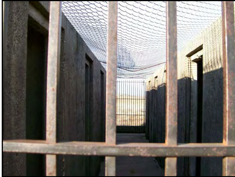
View Looking north into the Cell Block central hallway (Cheever/Berryman 2007) (Wire mesh covers top of the building)
