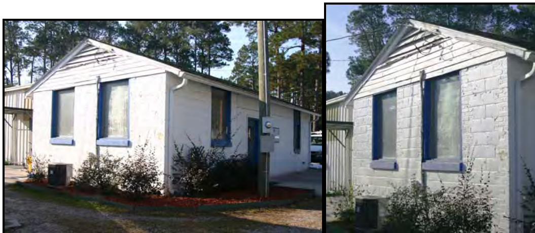
Building 5019 (Goodfellow 2007). Note the use of brickwork around the windows.
