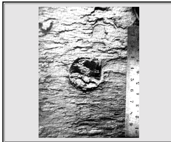
Figure 48. Peened end of rivet in Fig. 47 and exterior surface of hull plating (sandblasted). (Naval Research Laboratory)
