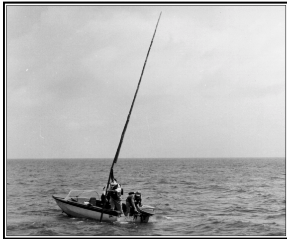
Figure 34. Long poles were used as reference guides for the dredge operator. (Smithsonian Institution)
