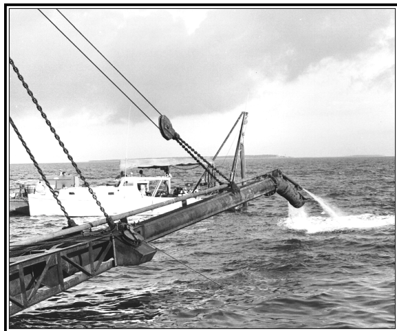
Figure 36. Dredge arm with twin water jets. (Smithsonian Institution)
