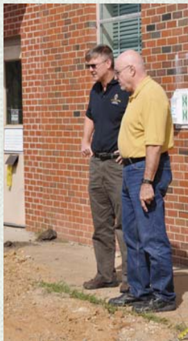
DLA Installation Support Project Manager Marvin Lockey (right) shows Damon Igou, installation energy manager, where wells were recently drilled to install ground source heat pumps.
