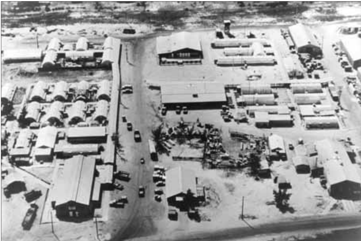
Naval Support Activity Hospital, Danang under construction in 1966.
