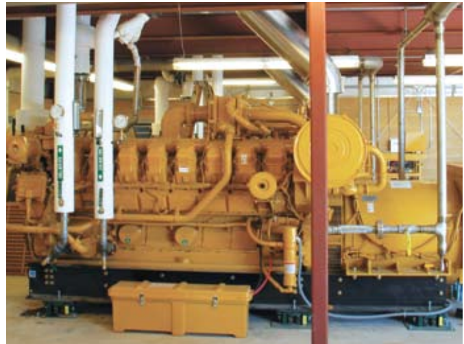
The DoD's first methane gas-to-energy generator at Hill Air Force Base produces energy by capturing gas from landfills.
