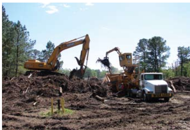
Heavily wooded sections of landfills were cleared, ground into wood chips and traded for compost.
