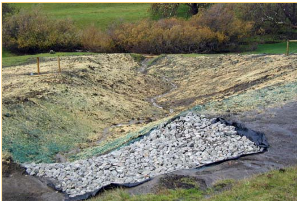
Problems at Dairy Creek were solved using bank stabilization techniques.
