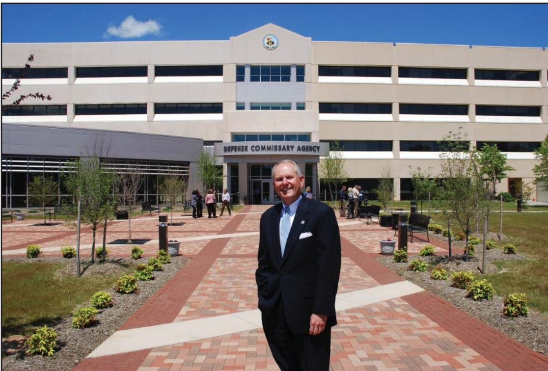
▲ HEADQUARTERS RENOVATION: Philip E. Sakowitz Jr., DeCA director and CEO, welcomes everyone to the headquarters building addition, Fort Lee, Va. New construction includes the wing left of the new central entrance area. The expansion makes room for DeCA employees currently working at the "Nic II" building in Hopewell. DeCA photo: Pete Skirbunt
