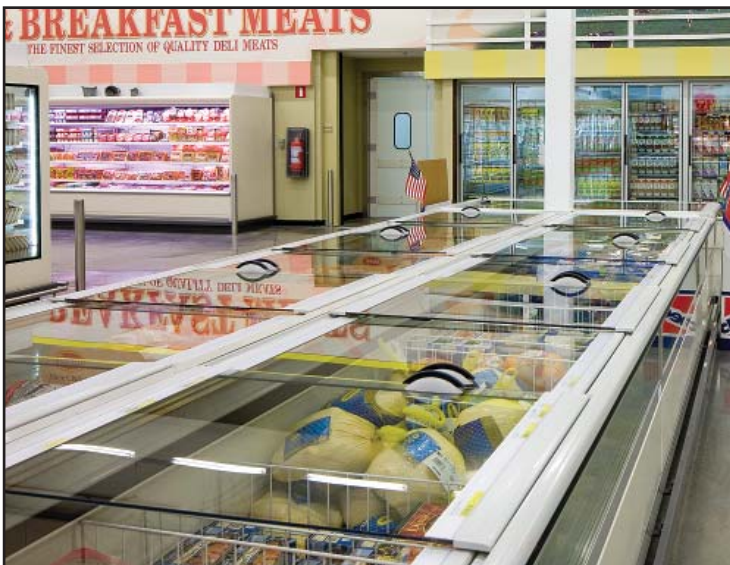
These enclosed, energy-efficient freezers, a low-profile style commonly called “coffin” cases, are built to European specifications and are not available in the United States. Coffins require more space than upright freezers but are thought to give customers a better line of sight to product assortment. DeCA photo: wallyimages.com
