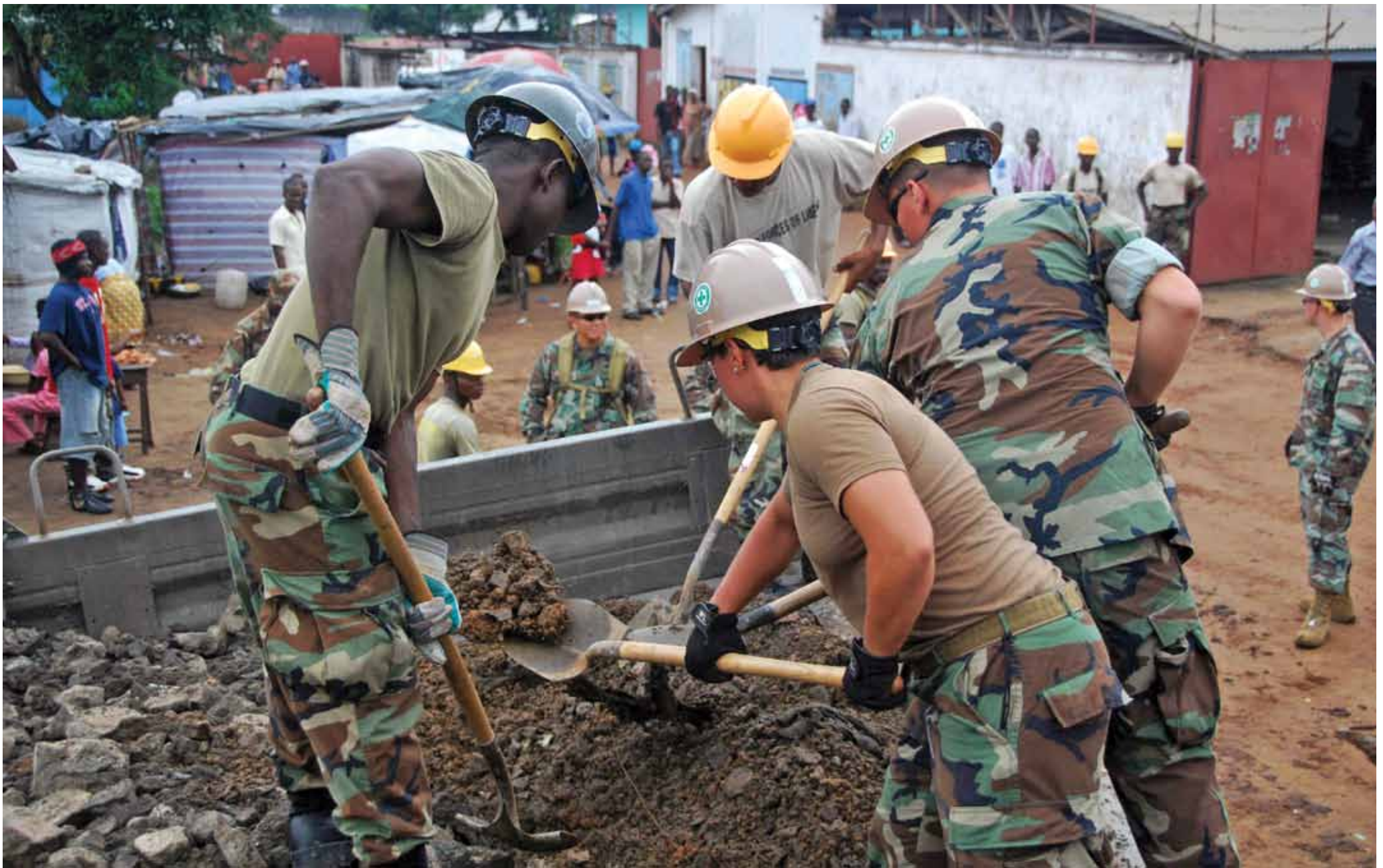
PEDIATRIC WARD - Armed Forces of Liberia (AFL) and U.S. Navy Seabees from Naval Mobile Construction Battalion (NMCB) 3 load dirt and debris into an AFL truck for removal from a building site at Redemption Hospital in Monrovia, Liberia, in September 2009. The personnel were building a pediatric ward and laundry facility as part of Africa Partnership Station. (U.S. Navy photo by Petty Officer 1st Class Dan Meaney)
