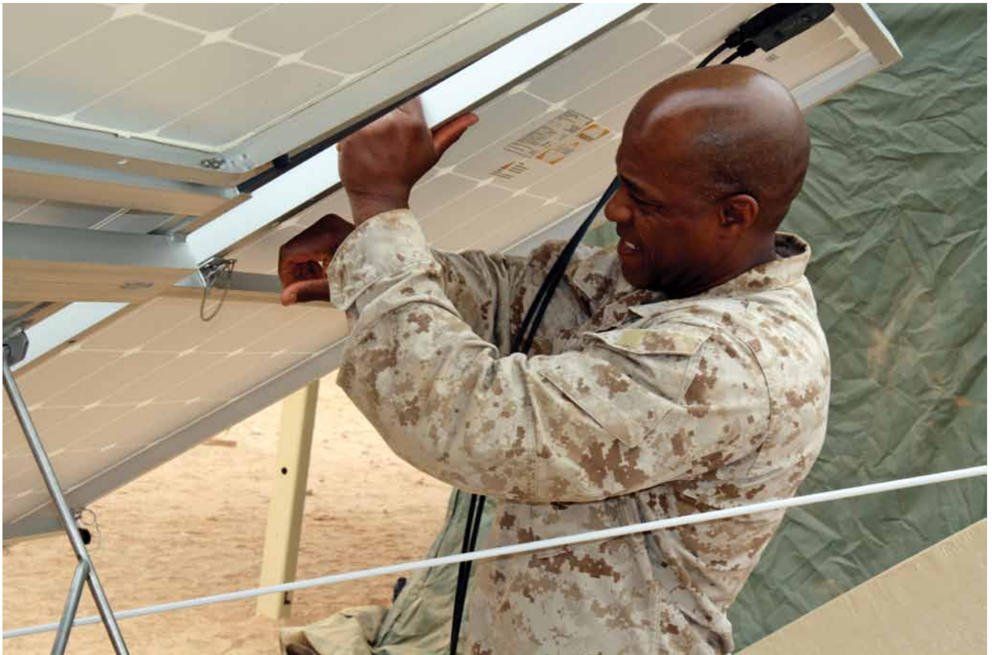
SUSTAINABLE ENERGY - Master Gunnery Sergeant Rowan Dickson locks down a solar panel in a power generating module for a test of the Expeditionary Forward Operating Base system during a testing and evaluation phase of Exercise African Lion 2010 at Tan Tan, Morocco, in May 19, 2010. The new environmentally-friendly energy system would enable deployed troops to purify water, light their tents and power their equipment through solar energy. It was tested in conjunction with African Lion, a AFRICOM-sponsored exercise involving more than 700 people. (U.S. Marine Forces Africa photo)
