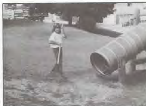
(Above) Adrienne Coll finishes leveling the filled-in pit at the base of one of the tunnel slides.
