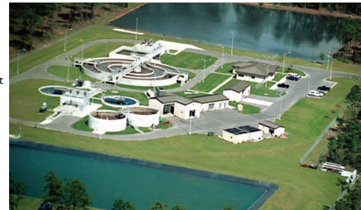
Hurburt Field, Florida Advanced Wastewater Treatment Plant.
