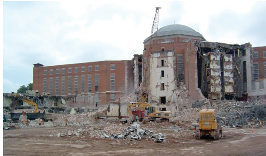
Demolition of Disciplinary Barracks at Fort Leavenworth, KS.
