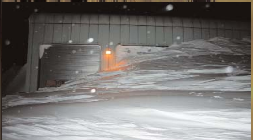
The February storm had 190 - 200 mph winds or higher. Roofs were peeled away and in one building, something pierced through the wall. The doors in are huge industrial garage doors, so the drift in that picture is immense.
