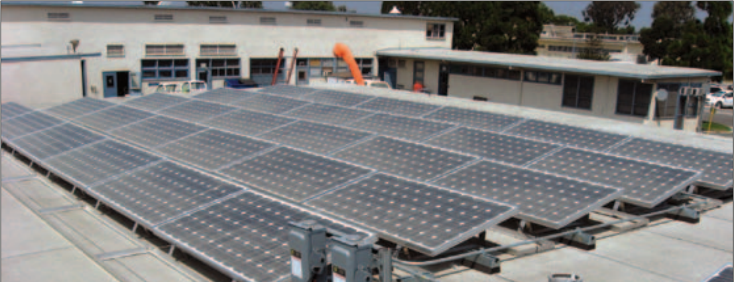
The California National Guard has adopted fuel cell systems powered by photovoltaic panels on some of their posts. These innovative hydrogen cells use a solar array to convert water into hydrogen gas through electrolysis and can be used to power various facilities. (Photo courtesy of the U.S. Army Environmental Command.)
