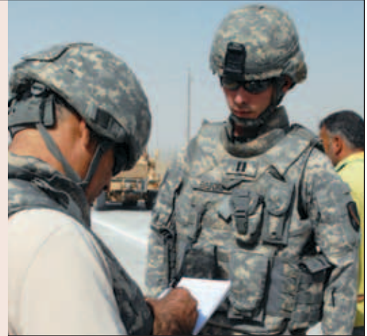
CPT Steven Belford, project manager for the 225th Engineer Brigade, briefs a DOD contractor during the final inspection before Maya Road in Baghdad opens to military and Iraqi civilian traffic. (U.S. Army photo by LTC Patrick Simon.)
