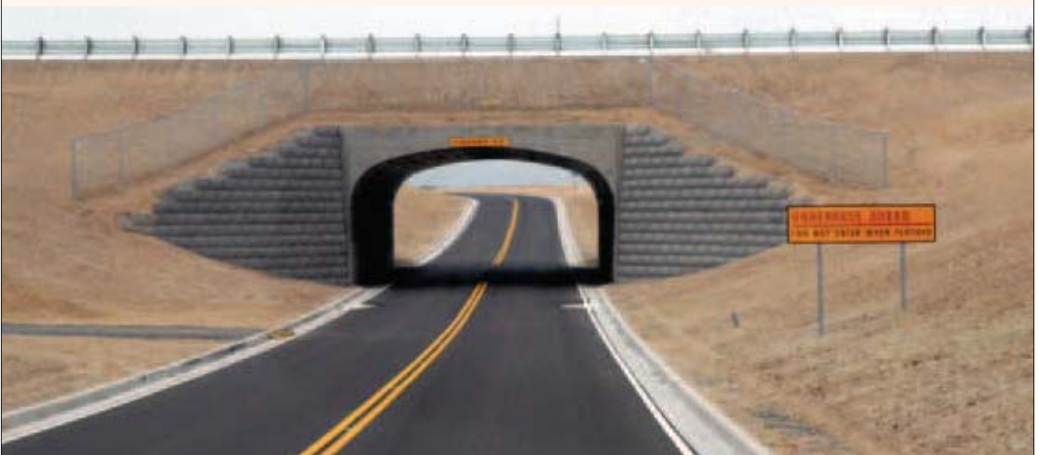
On the other side of this overpass is the ride and handling track, which has intentional defects ranging from mildly annoying tar strips and short waves to multiple waddles and deep troughs that bounce the stomach into the throat. The overpass is one of two circular tracks that simulate freeway driving. (U.S. Army photo by Mark Schauer.)
