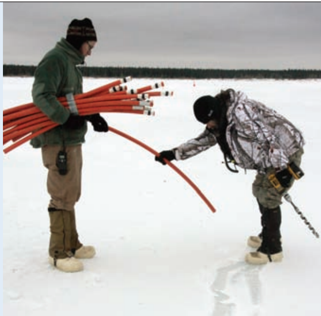
CRTC workers carefully mark the sides of the ice bridge to prevent drivers from mistakenly venturing off the carefully prepared bridge surface. (U.S. Army photo by Mike Kingston.)
