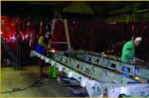
Then: The old process to grind and weld the FRS Flatrack was performed manually on saw horses and the operator needed to get in the right position. The operator was not able to move the weldment to the right height or ergonomic position. (Photo courtesy of RIA JMTC Lean Core Team.)
