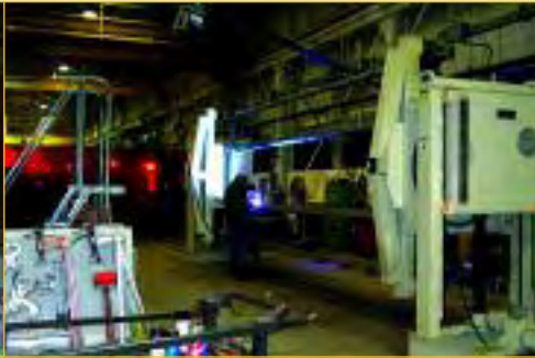
Now: The new grinding and welding process enables operators to use manipulators to easily rotate the weldment to the weld position and proper ergonomic height. (Photo courtesy of RIA JMTC Lean Core Team.)
