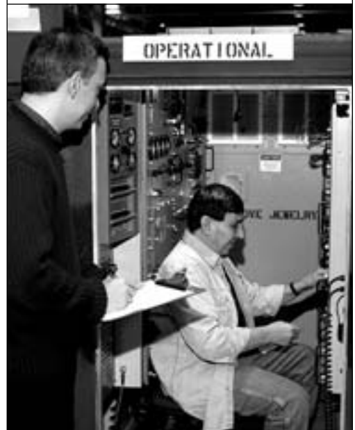
Don Engel (standing) collects data as Pete MacKarey, Communications Division Electronics Mechanic, Communications Systems Directorate, performs an azimuth and elevation adjustment on an AN/TRC-170 V3 alarm monitor. Engel is completing his black belt training and certification under a collaborative program sponsored by AMC. (U.S. Army photo by Anthony Medici.)
