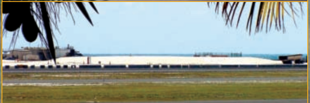
Johnston Atoll chemical disposal facility before and after dismantling and environmental remediation. (Photo courtesy of CMA.)
