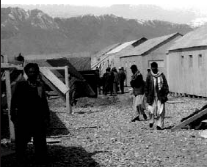
CCOs and MPs from the Bagram Contracting Office pay workers for building living quarters for coalition forces. (U.S. Army photo by MSG Bentura Fernandez.)
