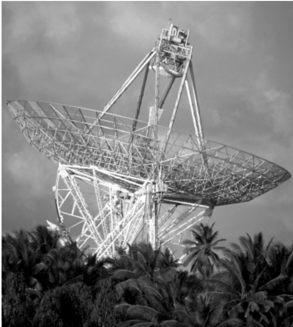
The ARPA Long Range Tracking and Instrumentation Radar, or ALTAIR, is one of four highly sophisticated radar systems at the Reagan Test Site being modernized with COTS equipment and software.
