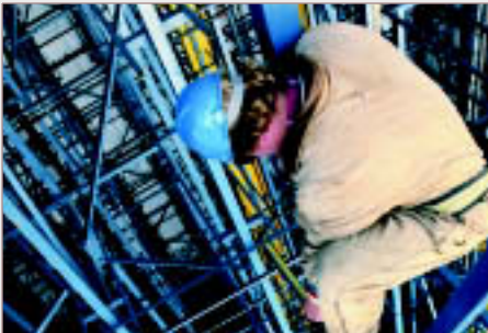
⑤ Structural metalworkers
