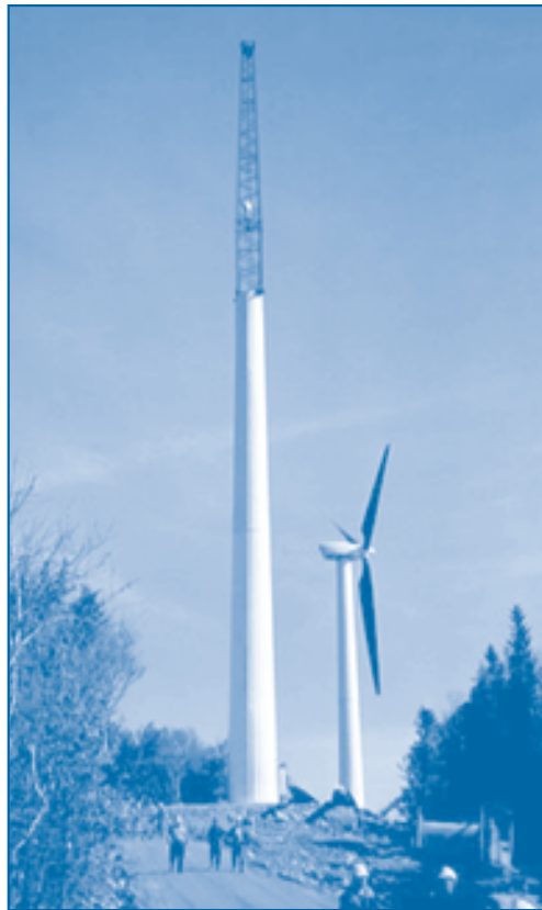
Wind Farm Under Construction
