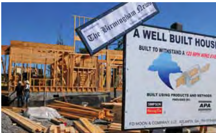
A house demolished by a tornado in Pratt City, Alabama, on April 27, 2011, gets rebuilt using construction methods that can withstand 120 mph winds.
