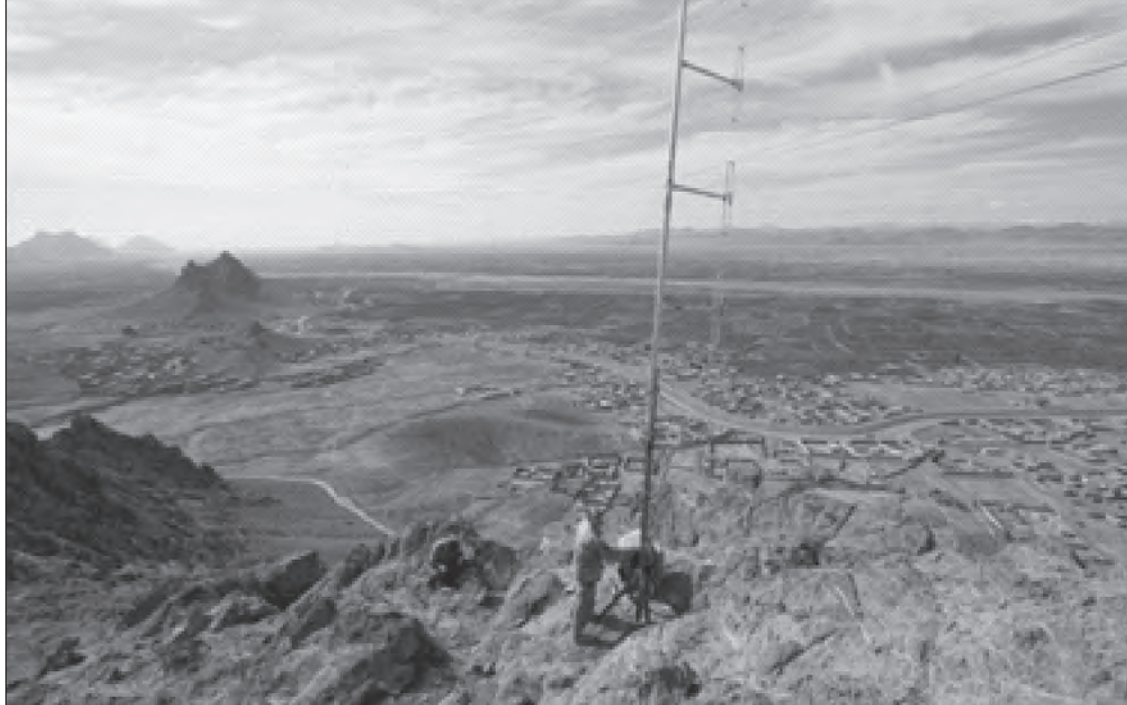
Antenna systems are installed to expand radio communications between the Arghandab District and Kandahar City.
