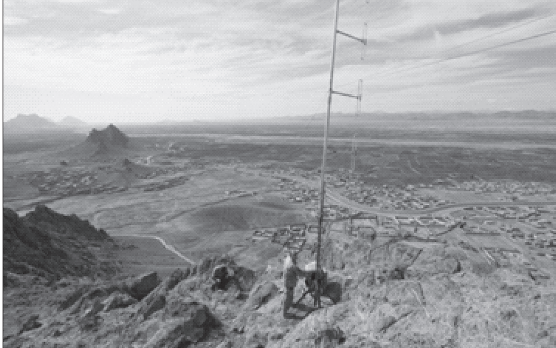
Antenna systems are installed to expand radio communications between the Arghandab District and Kandahar City.
