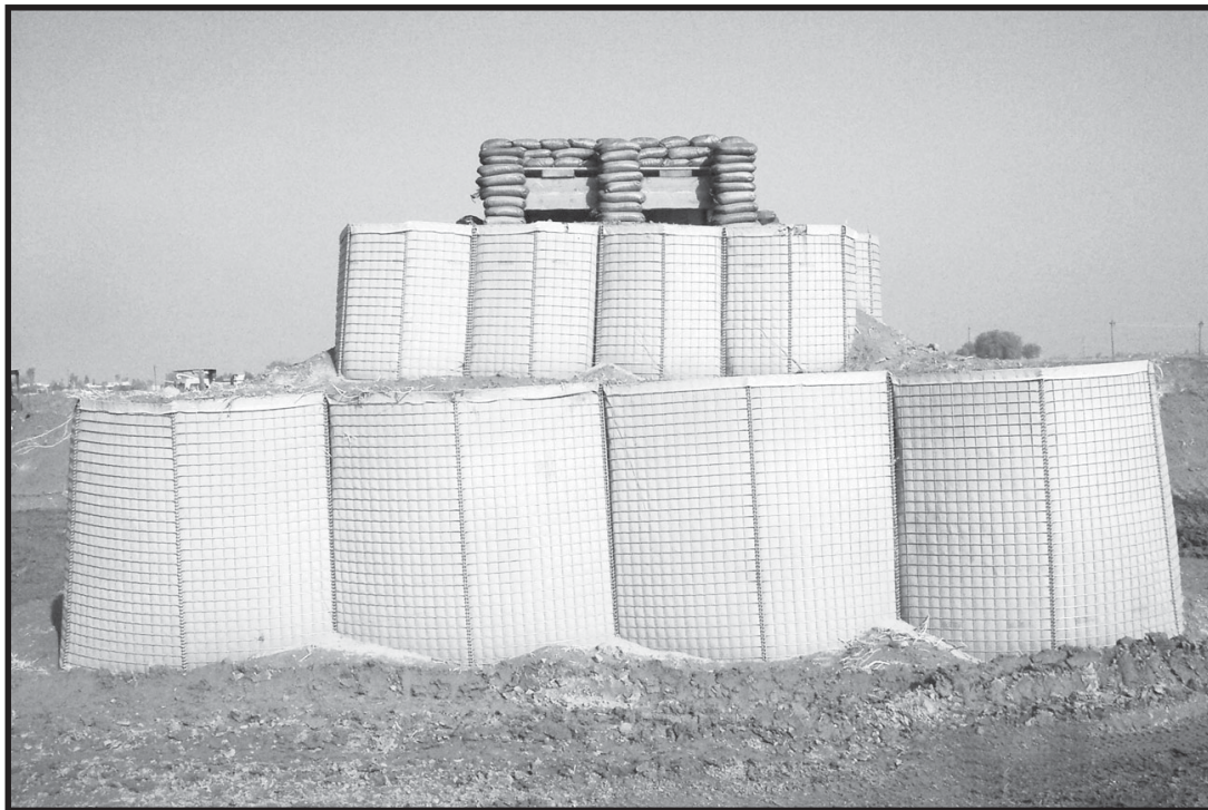
Hesco bastions topped with sandbags form a bunker and guard tower.
