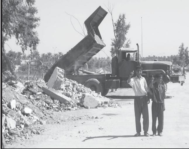
Rubble from demolition projects was reused to construct force protection berms.
