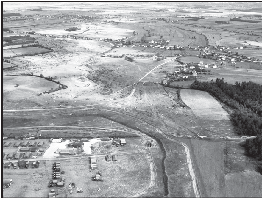
Advanced technologies will reduce site preparation time and logistics requirements, enabling support elements to keep pace with maneuver units.
