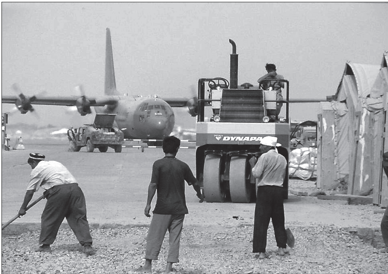
Road repair at K2 was a top priority in 2002 to improve theater logistics and airbase operations.
